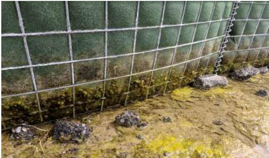
Notes: Moss is not a problem and does not cause any sort of accelerated degradation of the HESCO Bastion geotextile. It actually provides a barrier against UV rays and seems to be more beneficial than harmful.
