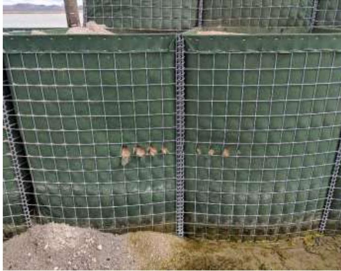
Notes: This is common form of damage where a vehicle or some sort of equipment 'side swipes' the HESCO Bastion and is generally not a huge issue. This can be repaired by overlapping another panel without even removing the damaged panel or by spraying/spackling a cement mixture over the holes.
