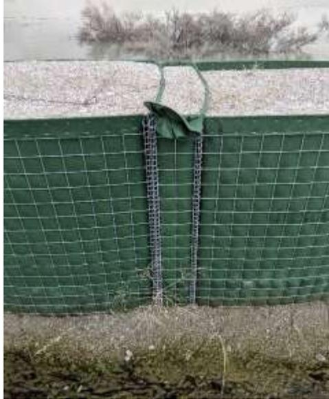
NOTE: This is likely were two sections came together and they took the time to modify a unit and create a good connection which was then correctly lined with geotextile.
