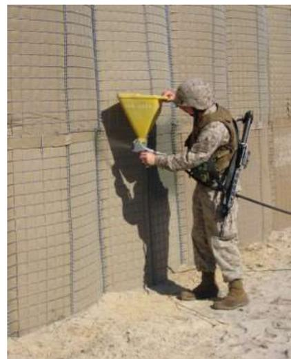
Picture: Cement Slurry for UV protection
