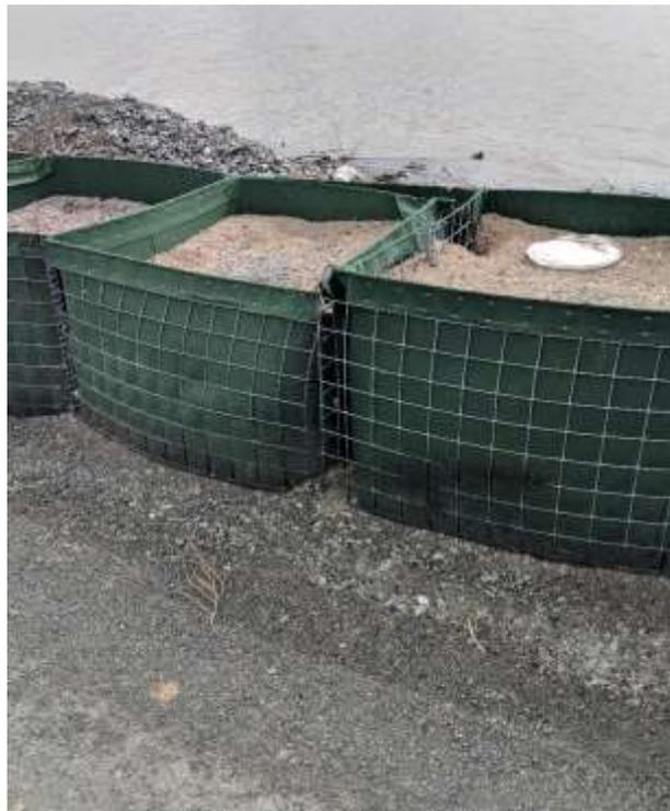
Notes: This is on the 'dry side' of the barrier and it would still function but I suggest you insert a coil to create a correct connection of the welded wire panels. Because the units are full, it may take a couple coils to tie it together.
