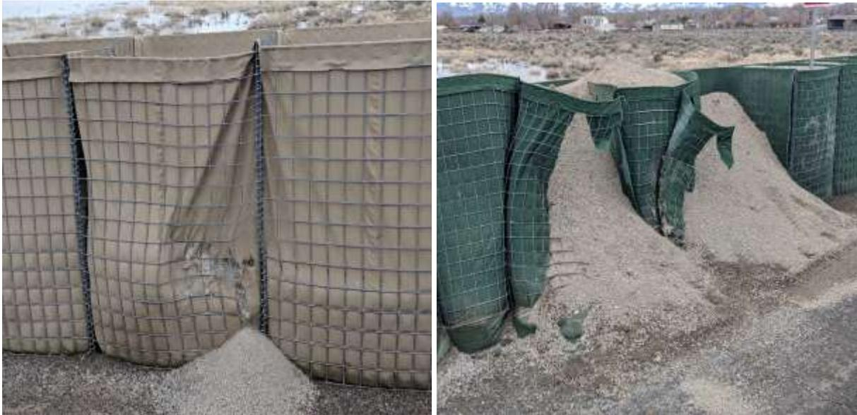
Notes: I viewed common damage associated with a vehicle impact. Repair as detailed above. The green units will require multiple panels and a pair of bolt cutters to cut the panels to fit the now deformed units.
