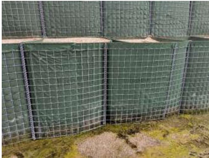
NOTE: It looks like someone missed inserting a joining pin during the initial layout and the units were filled. Someone in your staff identified this and overlapped it with two face panels AND figured out the lesser-known technique of screwing the coil to the weldmesh itself to create a fantastic fix. I really appreciate the attention to detail in taking the time to fix it!
