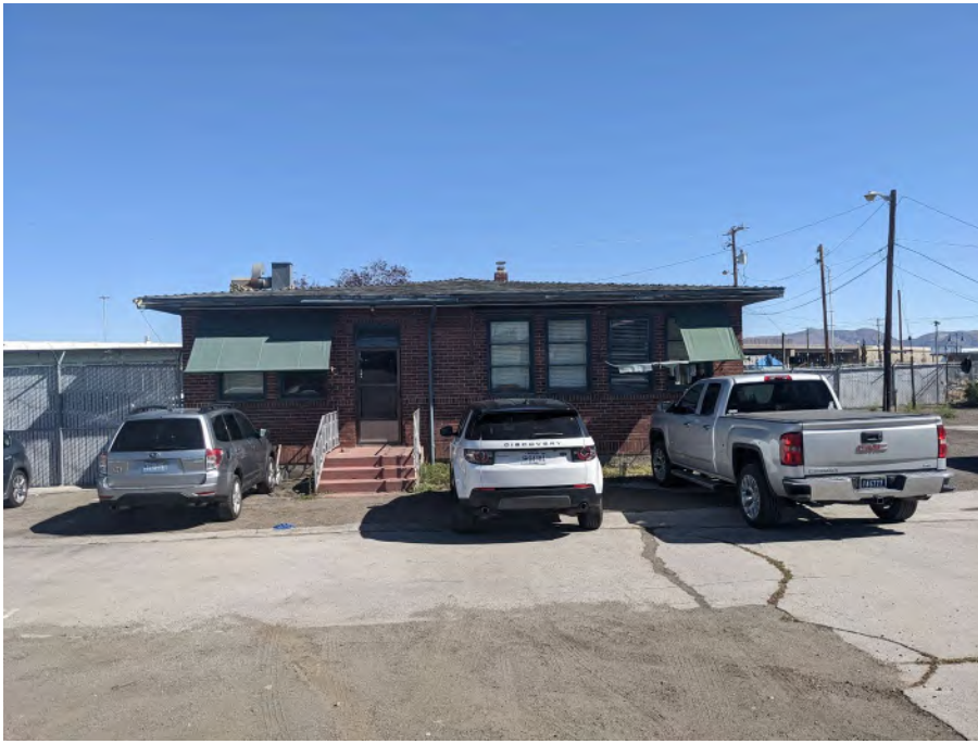
Elevation: B15585 Western elevation Direction facing: 90 Date: 10/4/2022
