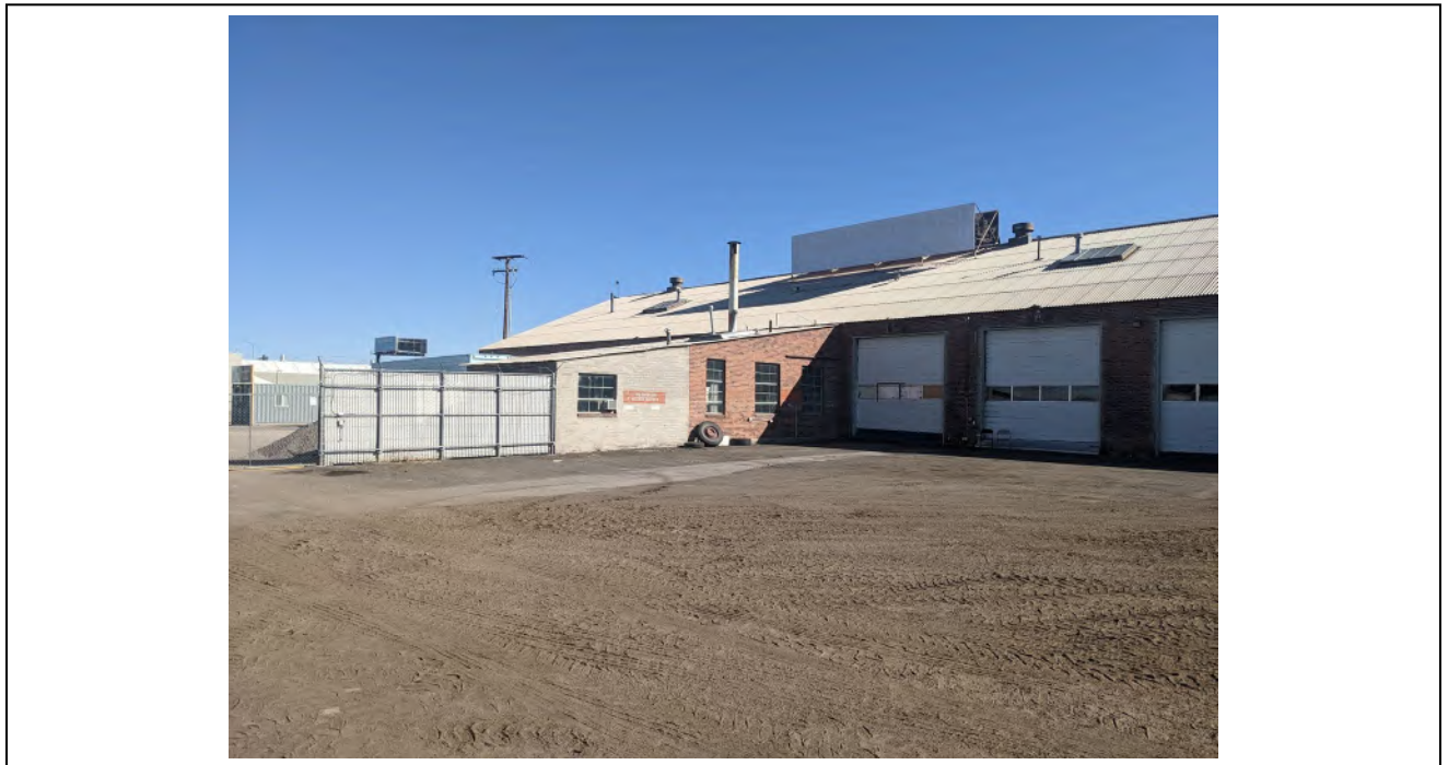
Elevation: Building 2 Boiler Room Date: 10/4/2022
