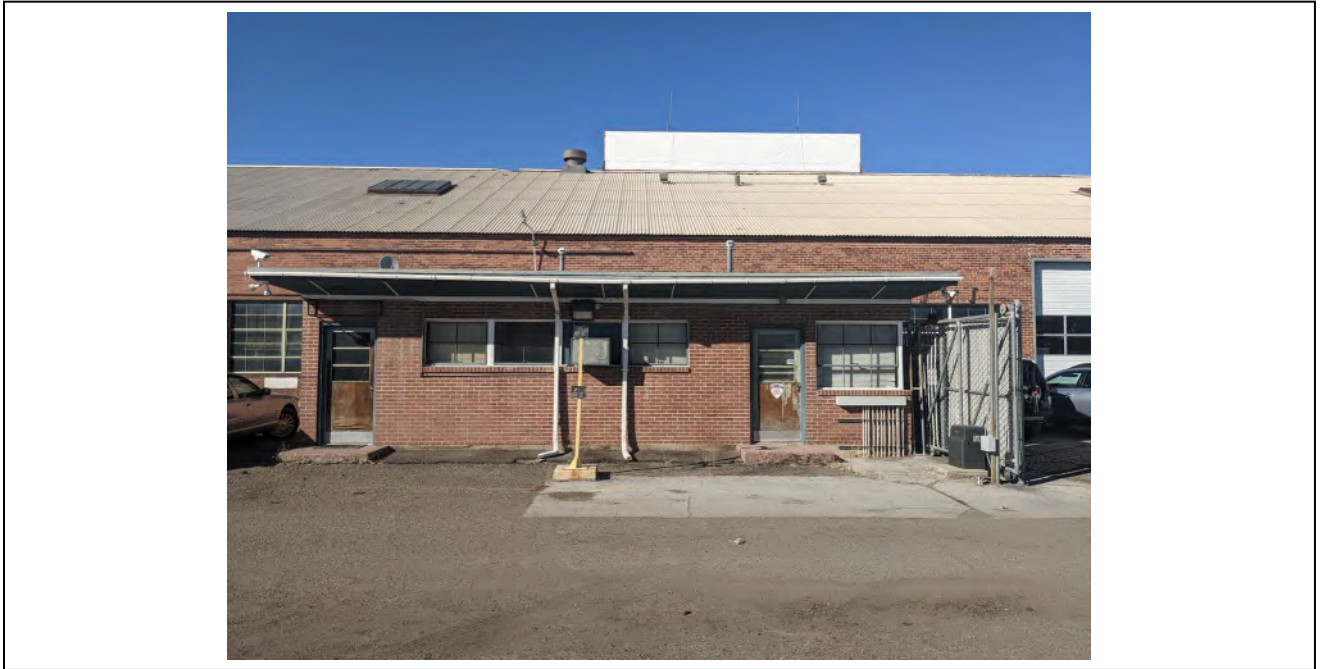
Elevation: Building 2 Front Wall Addition Date: 10/4/2022
