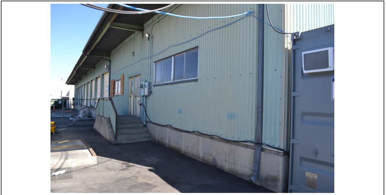
Elevation: Building 3 Main entrance Date: 10/4/2022
