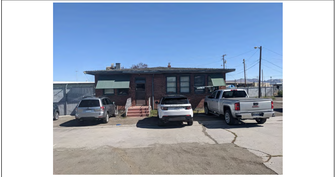
Elevation: B15585 Western elevation Direction facing: 90 Date: 10/4/2022
