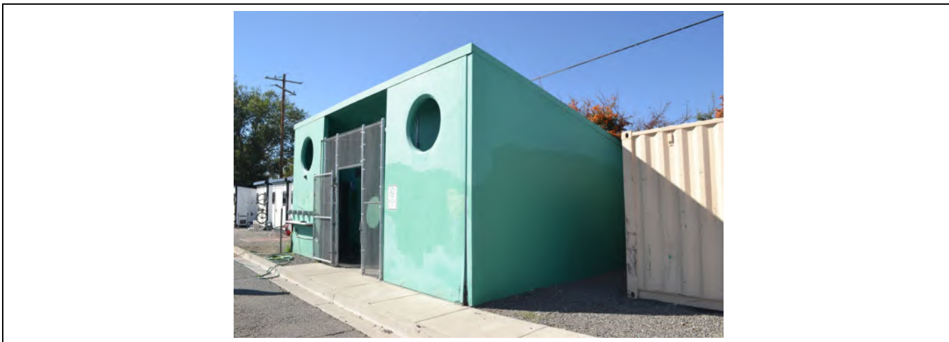
Elevation: Oblique view of restroom Direction facing: 210 Photographer: S Rathbone Date: 10/4/2022
