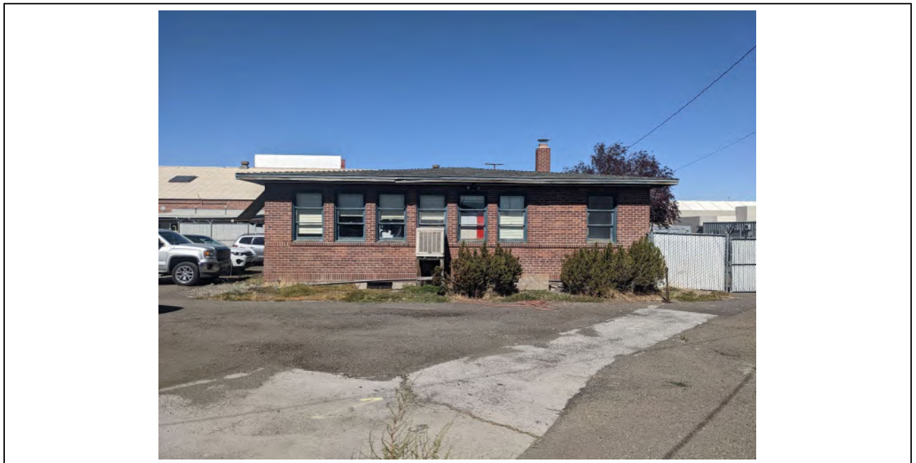
Elevation: B15585 Southern elevation Direction facing: 0 Date: 10/4/2022
