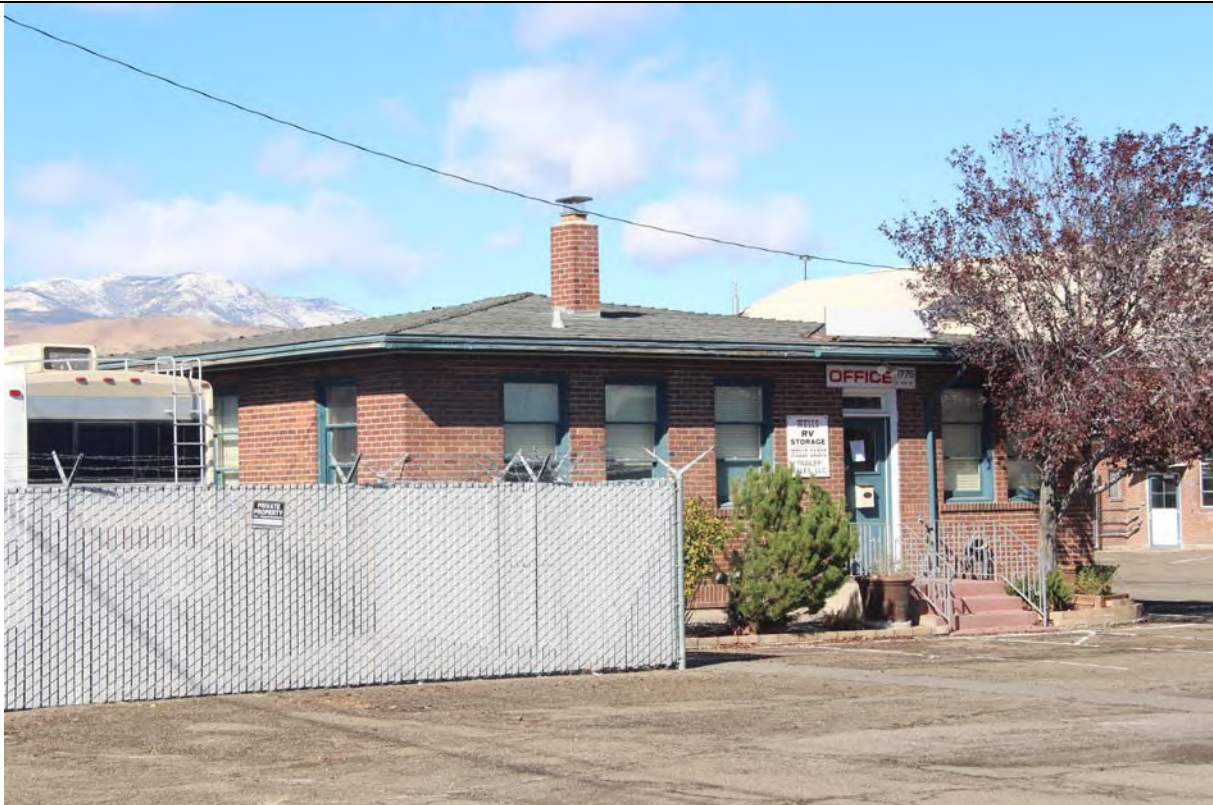
Elevation: east Direction facing: northwest Photographer: Mead & Hunt, Inc. Date: 10/20/2017
