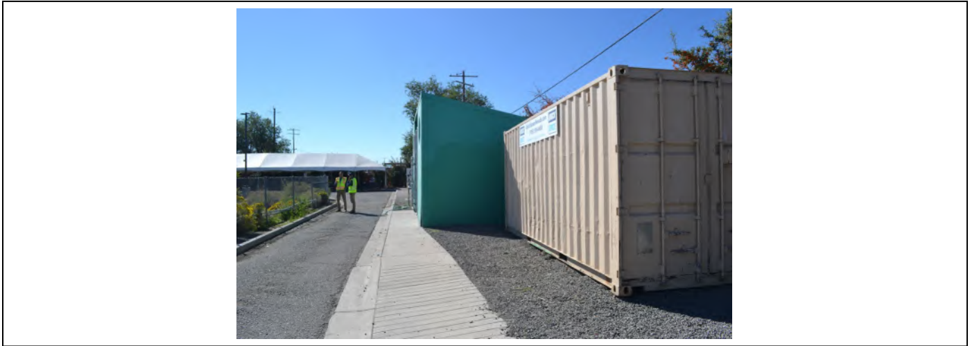
Elevation: Side elevation of restroom Direction facing: 180 Photographer: S Rathbone Date: 10/4/2022
