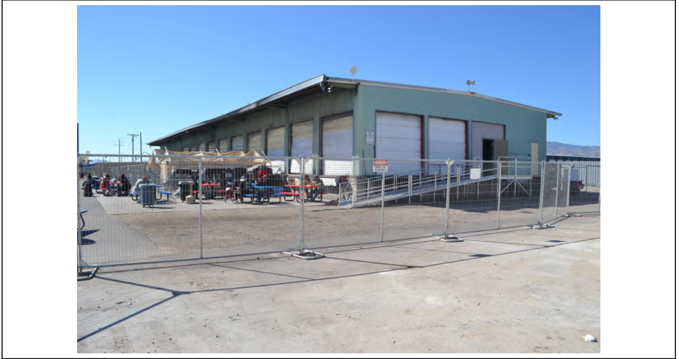
Elevation: Building 3 Northeast elevation Date: 10/4/2022
