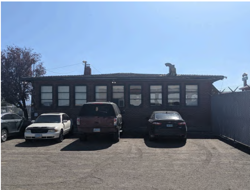
Elevation: B15585 Northern elevation Date: 10/4/2022
