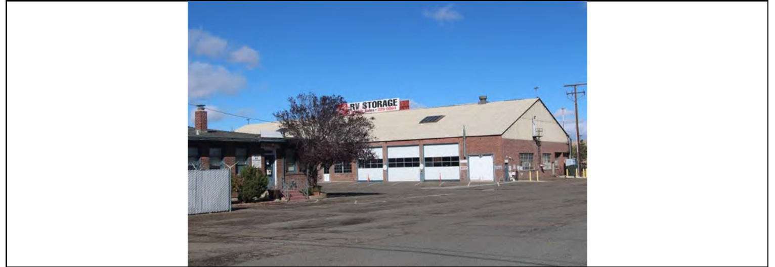
Elevation: south Direction facing: northwest Photographer: Mead & Hunt, Inc. Date: 10/20/2017
