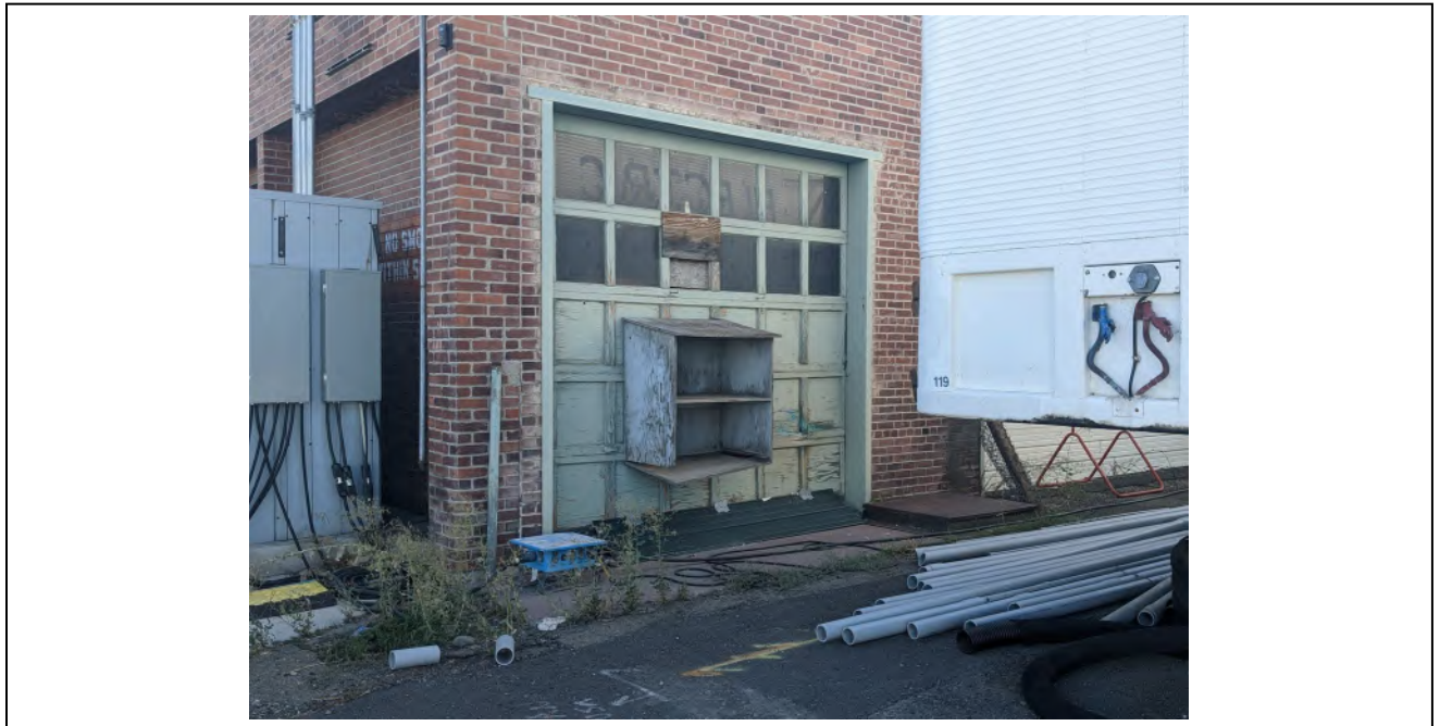
Elevation: Building 2 Door detail at east end of north wall Photographer: S Rathbone
