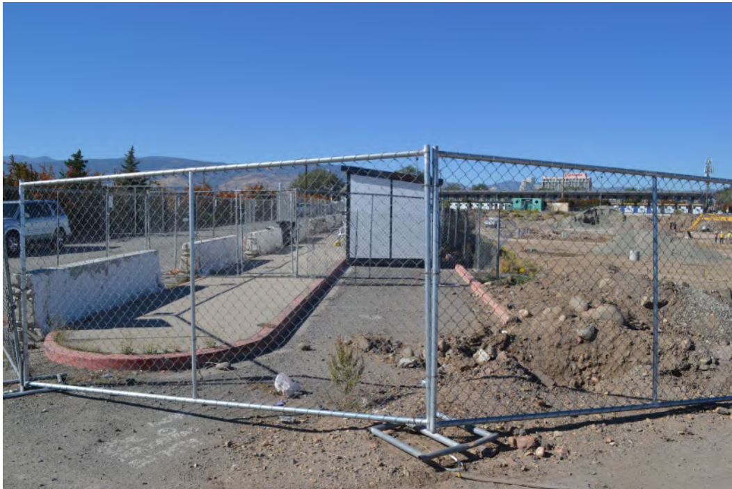
Elevation: Path running along the top of the bank to the northwest of Line Drive Direction facing: 240 Photographer: S Rathbone Date: 10/4/2022
