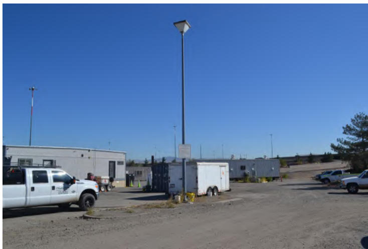
Elevation: Parking Lot floodlight Direction facing: 50 Photographer: S Rathbone Date: 10/4/2022
