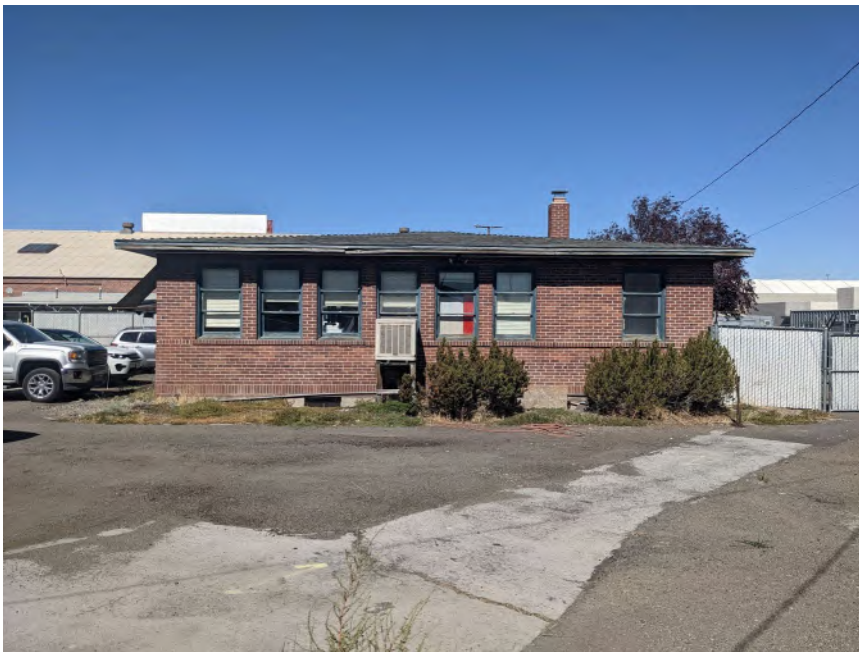
Elevation: B15585 Southern elevation Direction facing: 0 Date: 10/4/2022
