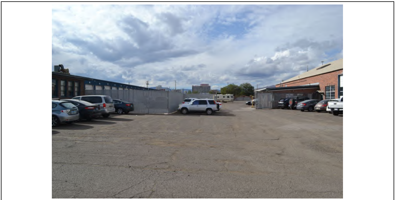
Elevation: Detail of Structure 3 running between B15585 and Building 2 Photographer: S Rathbone
