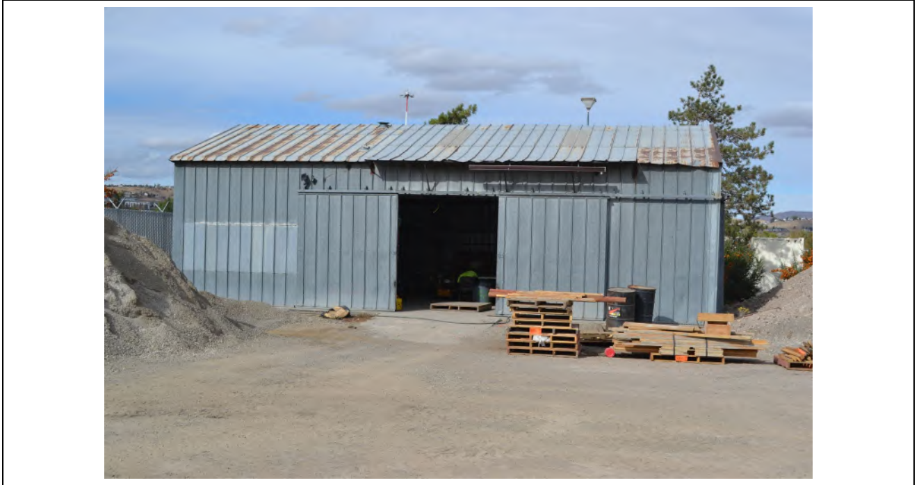
Elevation: Building 4 South elevation Date: 10/25/2022
