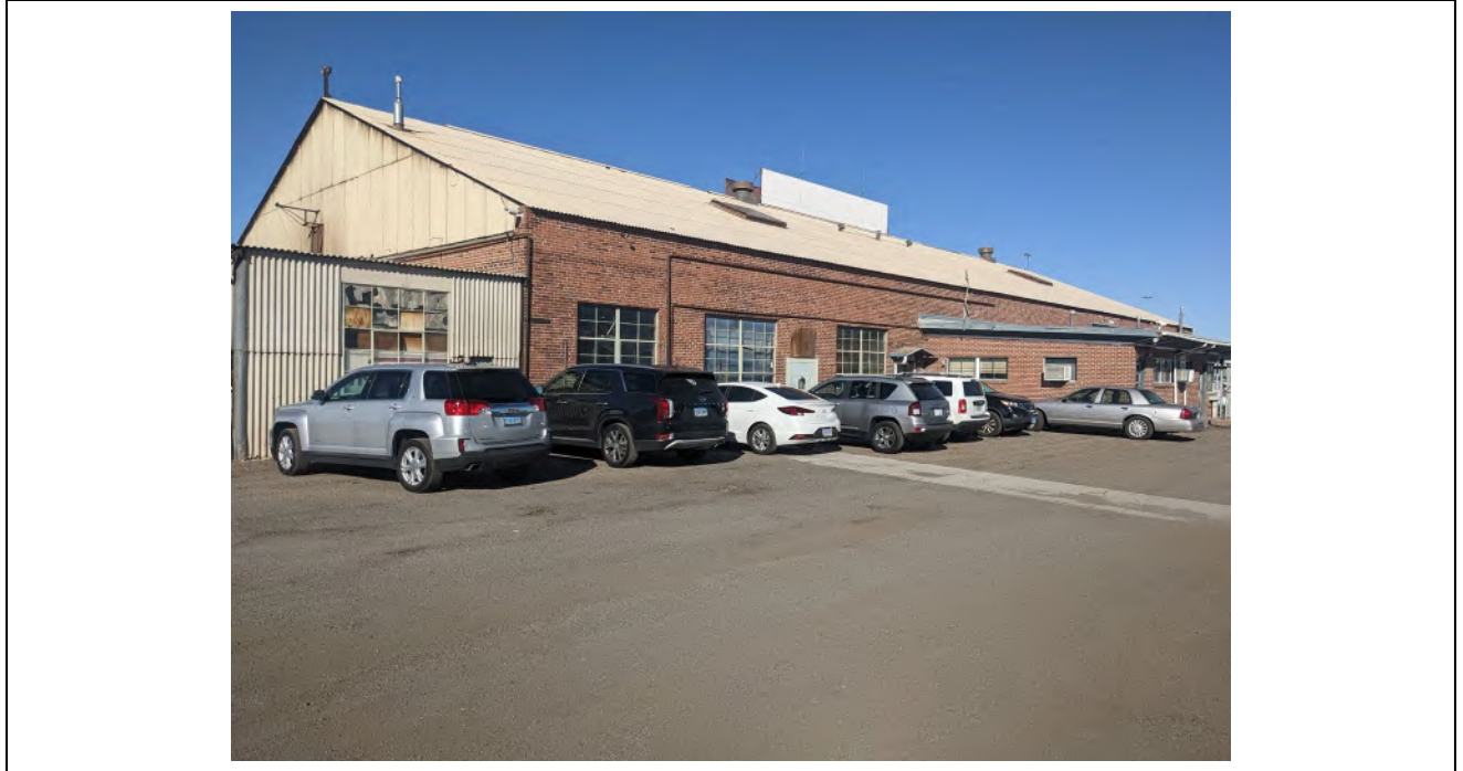
Elevation: Building 2 South elevation Date: 10/4/2022
