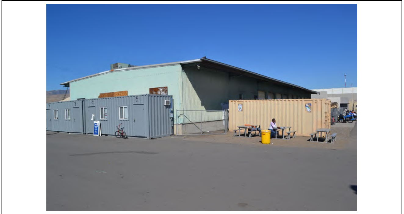
Elevation: Building 3 Southeast corner Date: 10/4/2022
