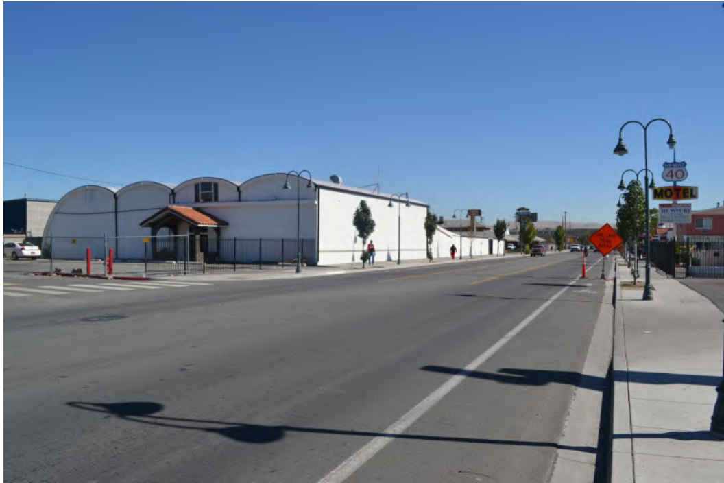
Photograph 13: View towards the project area from E 4th Street & Line Drive Direction facing: 50
