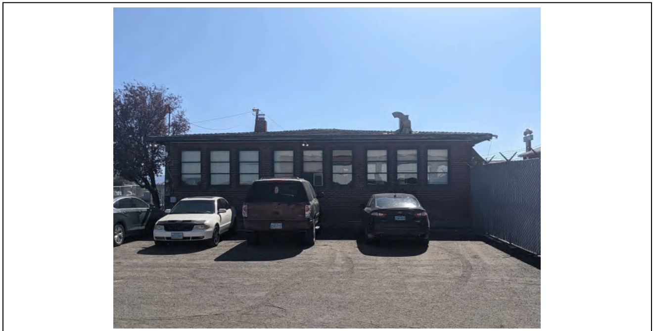
Elevation: B15585 Northern elevation Date: 10/4/2022
