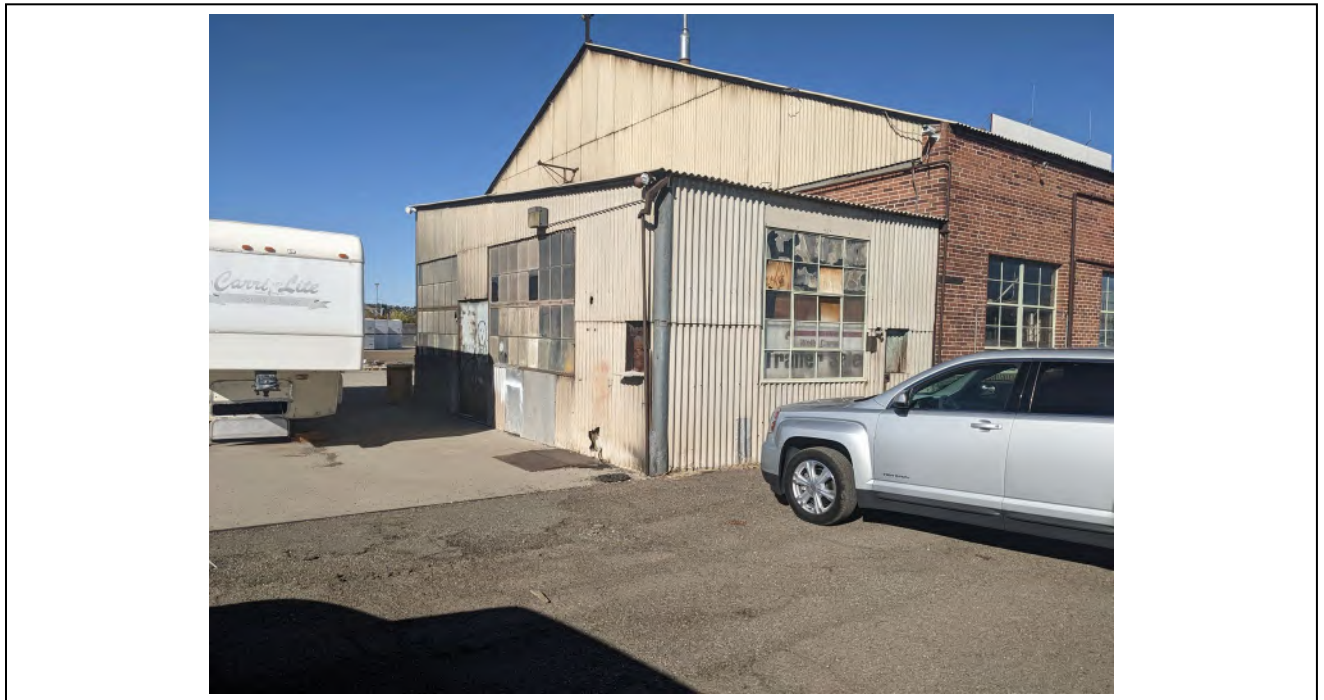
Elevation: Building 2 West Wall Addition Date: 10/4/2022
