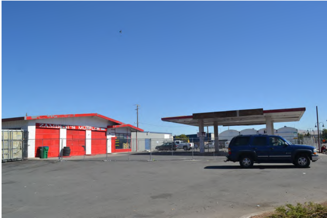
Photograph 11: View of Zamboni's Muffler with Project Area in the background
