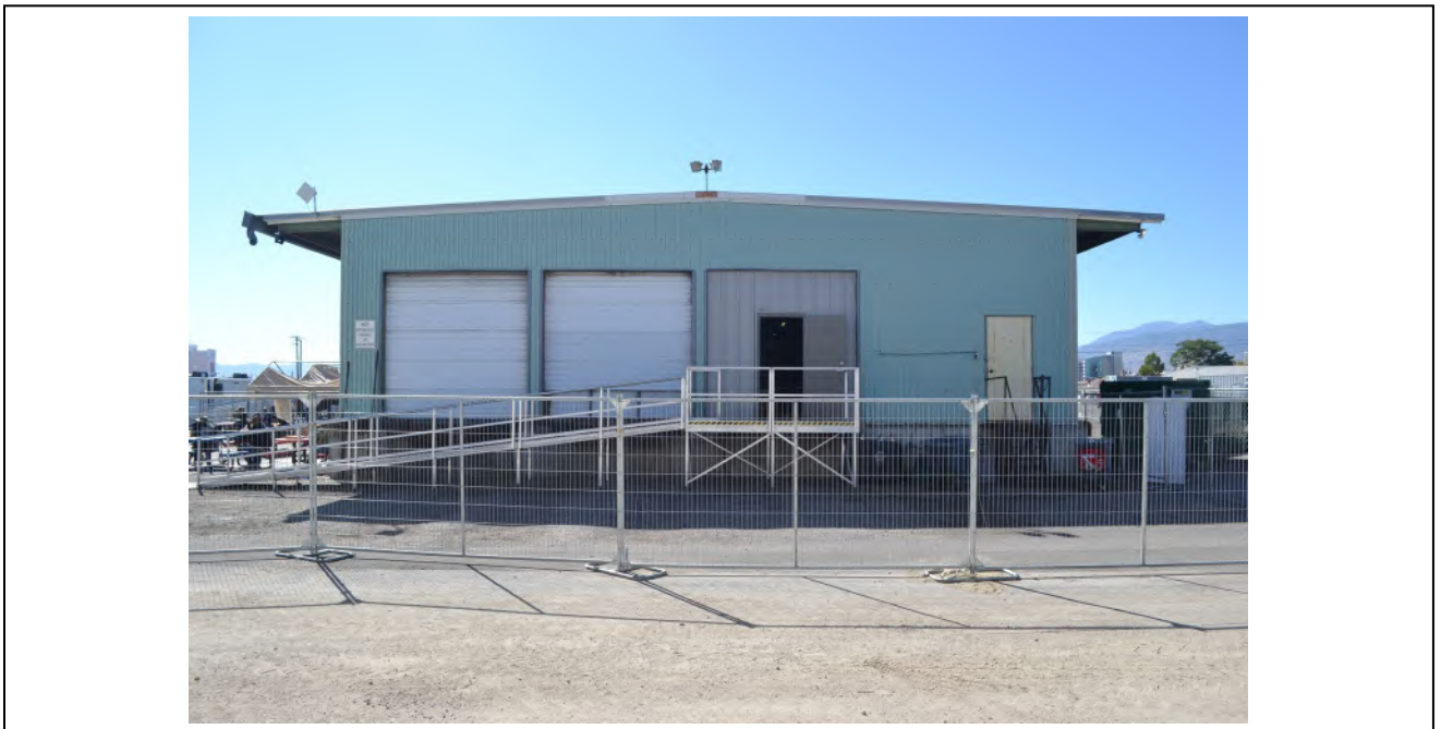
Elevation: Building 3 North elevation Direction facing: 180 Date: 10/4/2022
