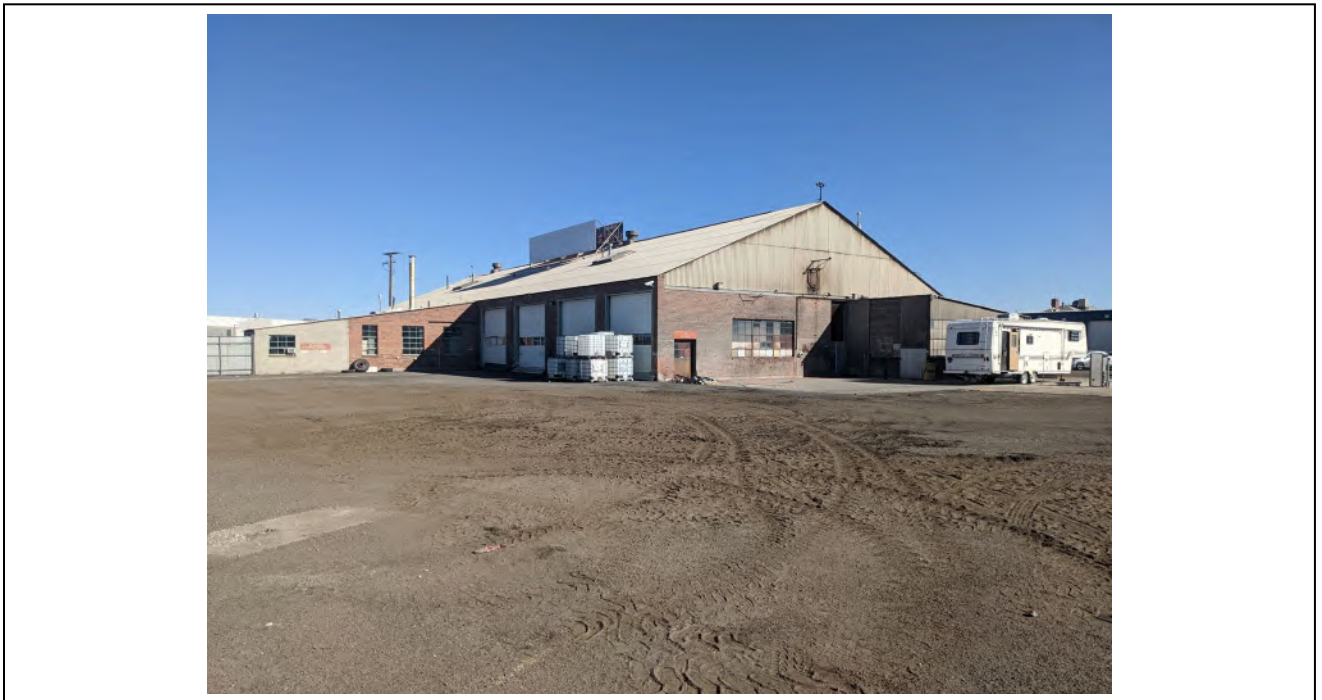
Elevation: Building 2 North west corner Date: 10/4/2022
