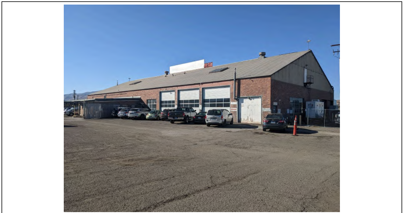
Elevation: Building 2 South elevation Date: 10/4/2022
