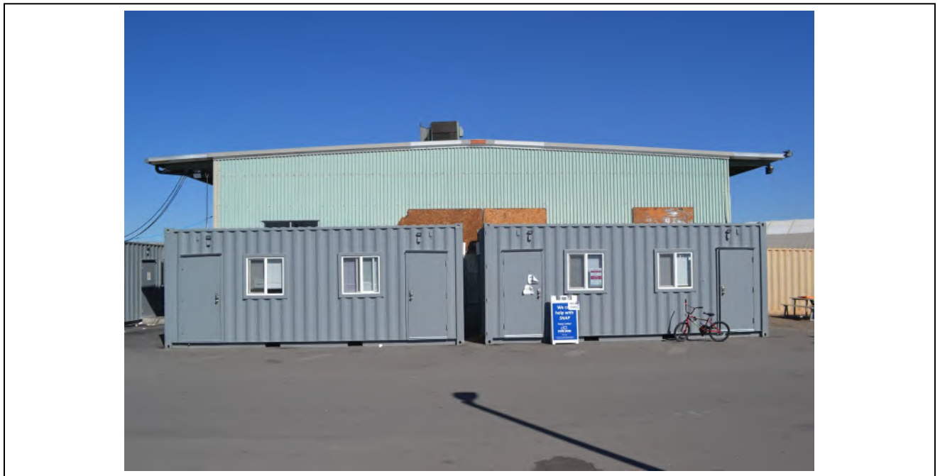
Elevation: Building 3 South elevation Date: 10/4/2022
