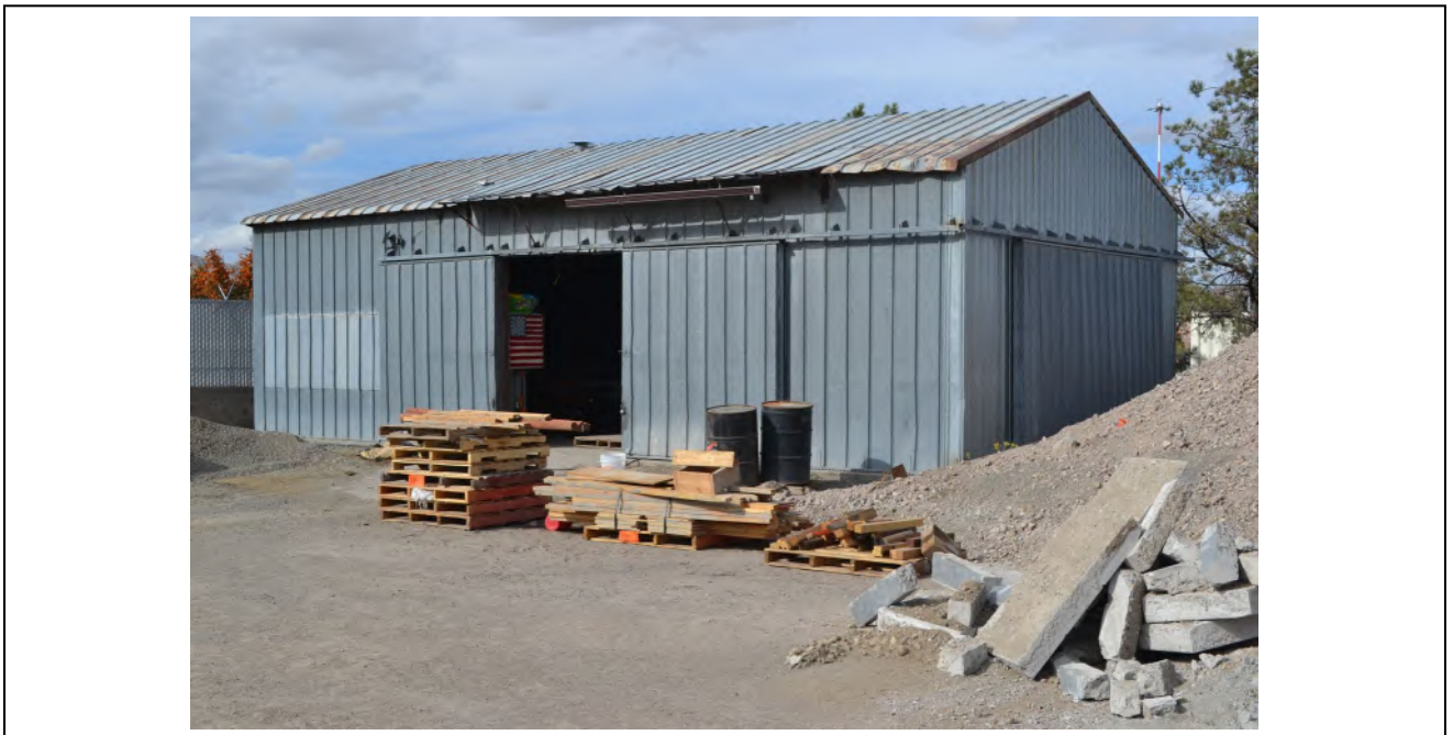
Elevation: Building 4 Southeast corner Date: 10/25/2022
