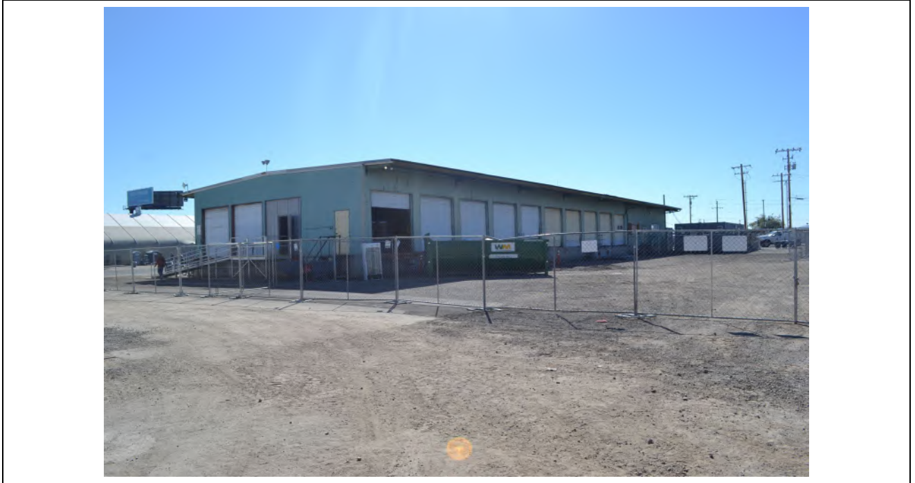
Elevation: Building 3 Northwest corner Direction facing: 130 Date: 10/4/2022
