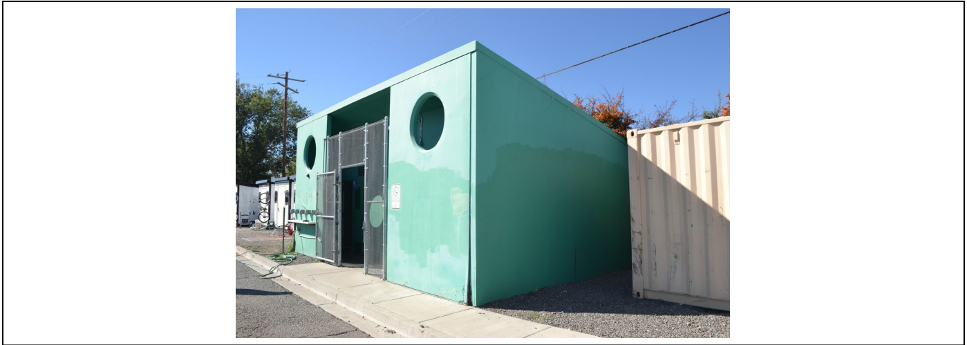
Elevation: Oblique view of restroom Direction facing: 210 Photographer: S Rathbone Date: 10/4/2022
