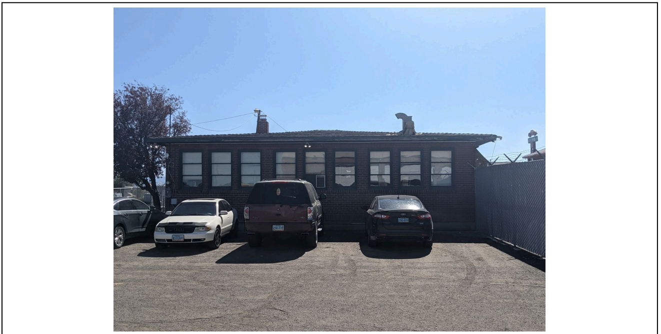
Elevation: B15585 Northern elevation Date: 10/4/2022
