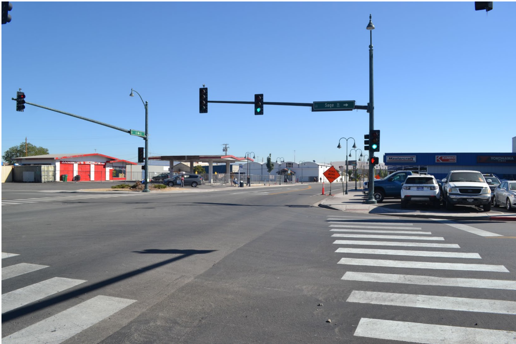
Photograph 10: View towards the project area from E 4th Street & Sage Street Direction facing: 80
