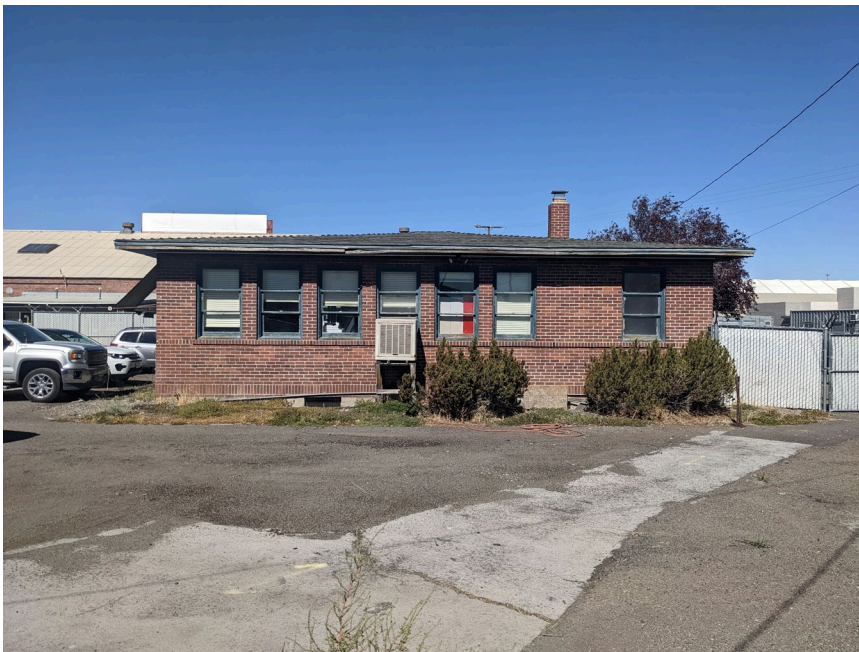
Elevation: B15585 Southern elevation Direction facing: 0 Date: 10/4/2022
