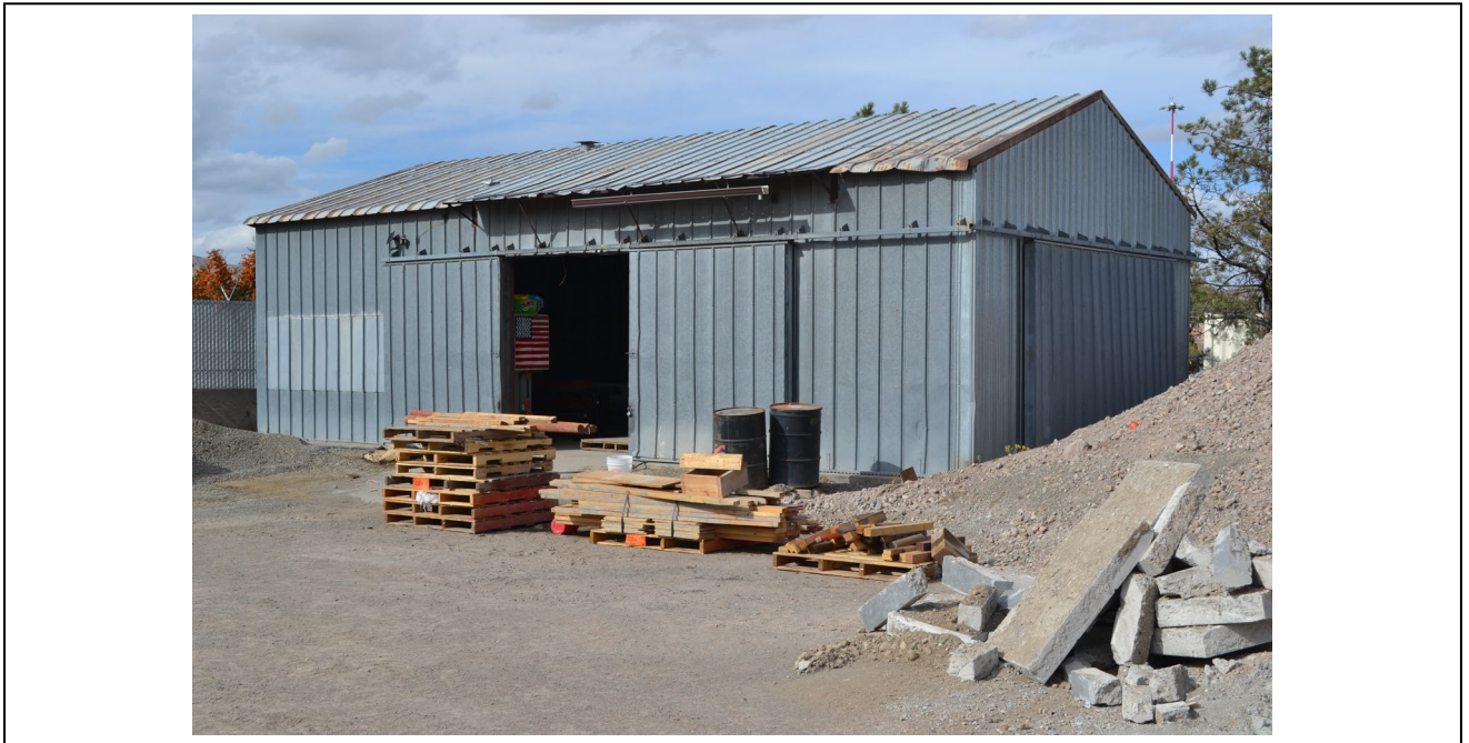
Elevation: Building 4 Southeast corner Date: 10/25/2022
