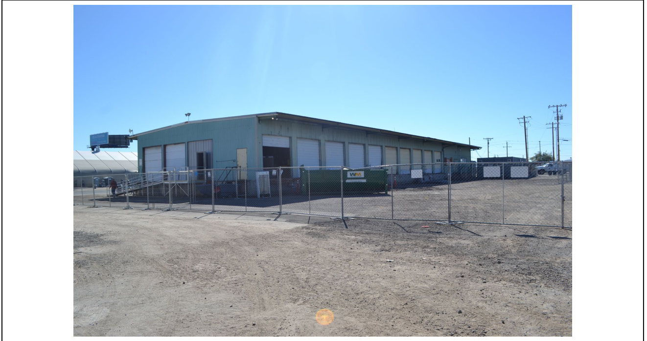
Elevation: Building 3 Northwest corner Direction facing: 130 Date: 10/4/2022
