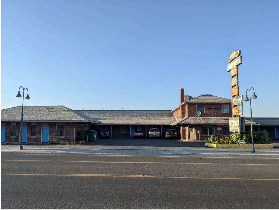
Photograph 17: View of Sandman Motel with Project Area in the background Direction facing: 0
