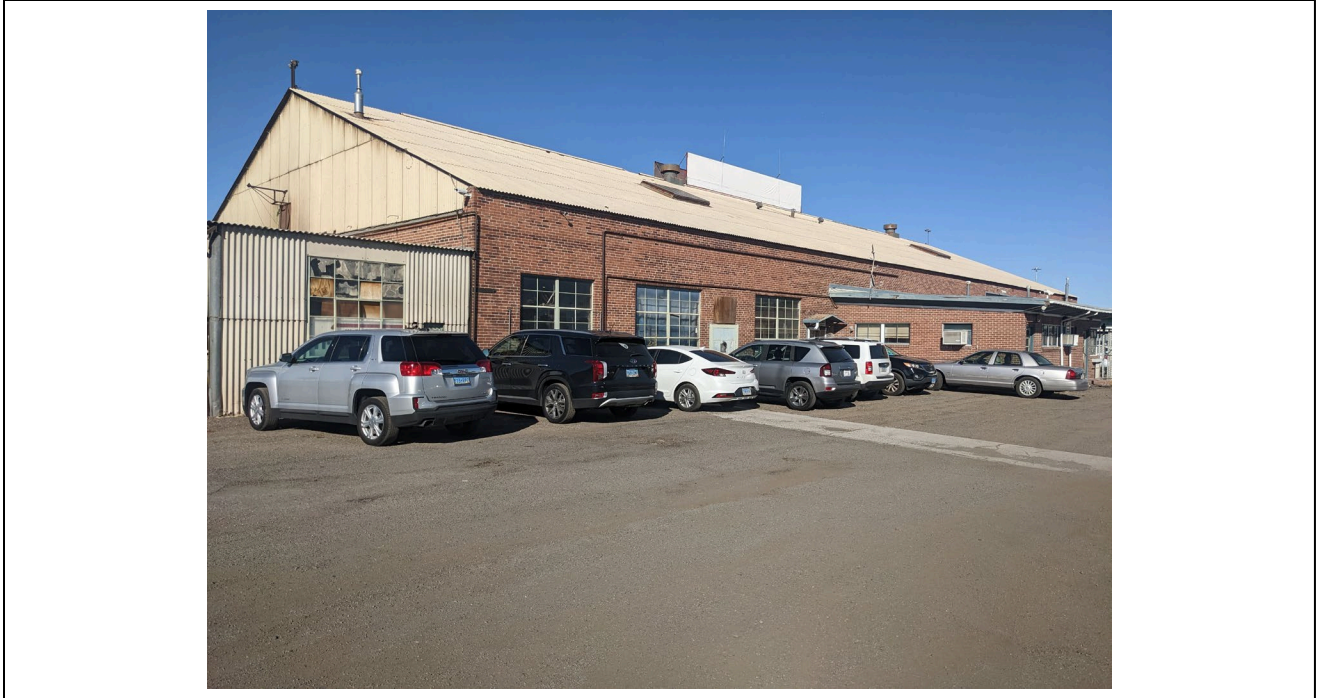
Elevation: Building 2 South elevation Date: 10/4/2022
