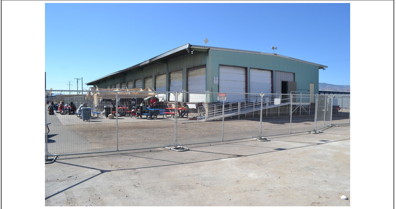
Elevation: Building 3 Northeast elevation Date: 10/4/2022
