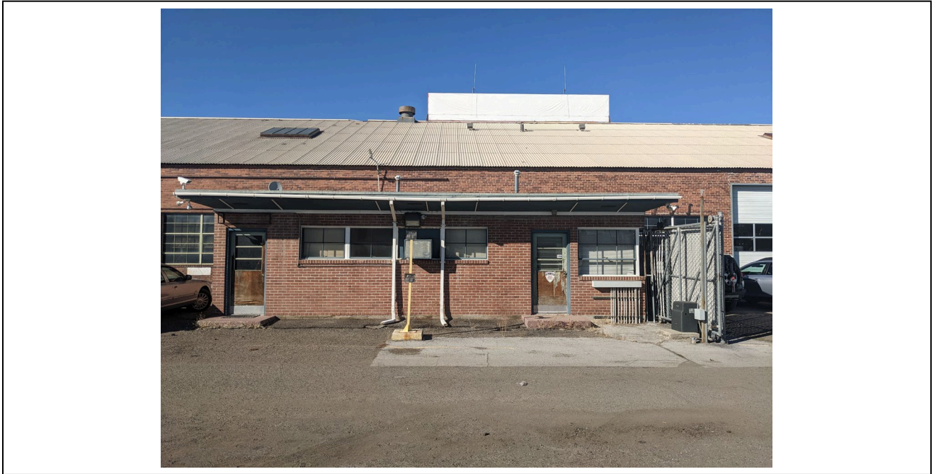
Elevation: Building 2 Front Wall Addition Date: 10/4/2022
