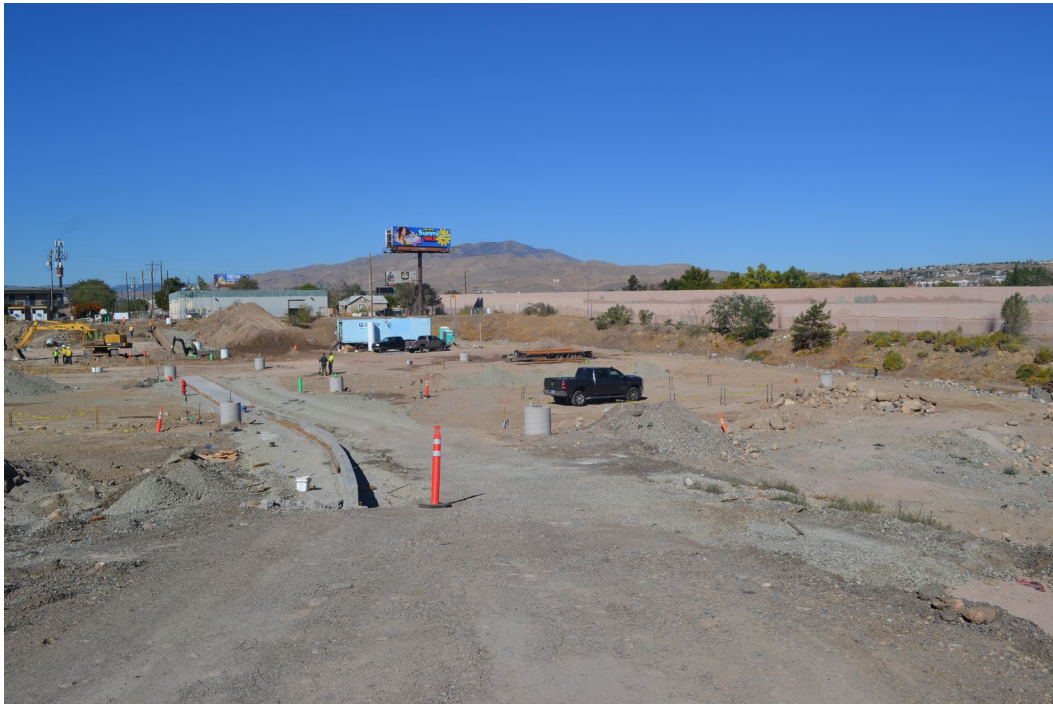
Elevation: Governor's Bowl Park construction site overview Date: 10/4/2022
