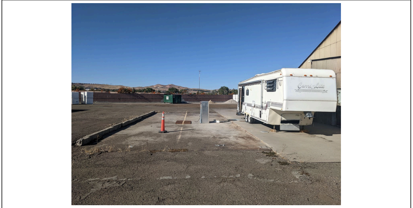
Elevation: Building 2 External Garage Foundations Photographer: S Rathbone
