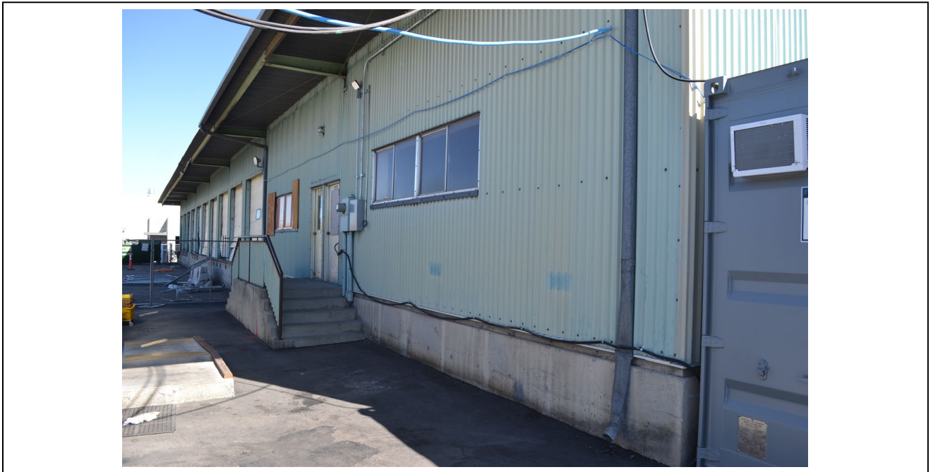
Elevation: Building 3 Main entrance Date: 10/4/2022
