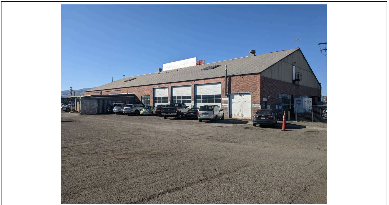
Elevation: Building 2 South elevation Date: 10/4/2022
