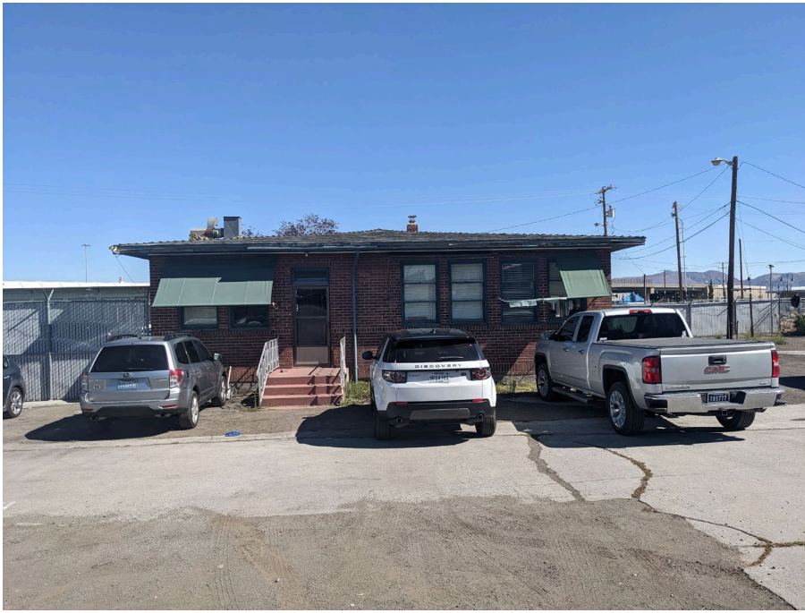
Elevation: B15585 Western elevation Direction facing: 90 Date: 10/4/2022
