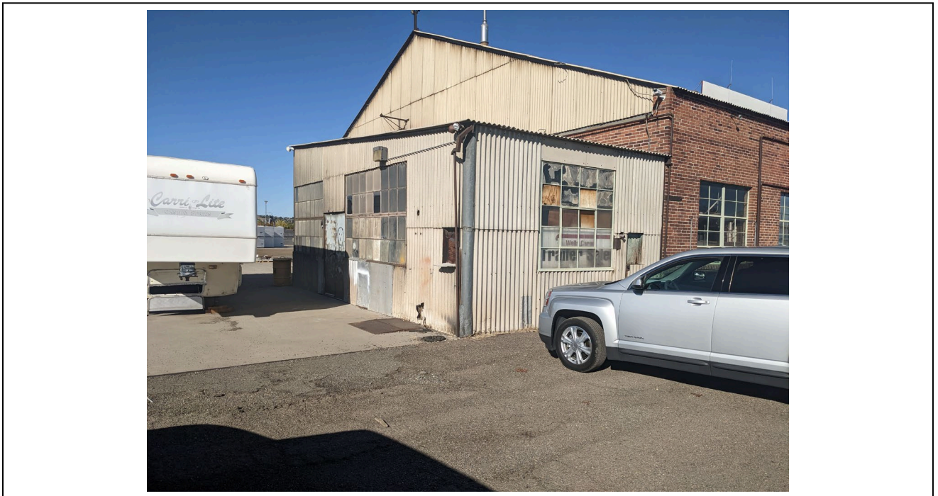
Elevation: Building 2 West Wall Addition Date: 10/4/2022
