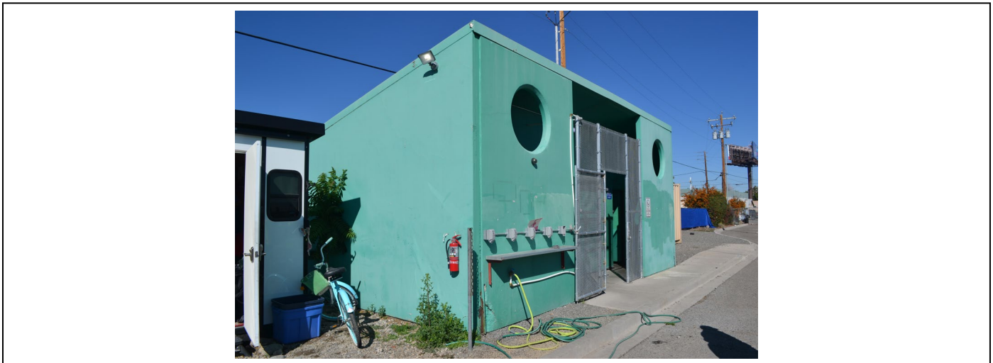
Elevation: Oblique view of restroom Direction facing: 320 Photographer: S Rathbone Date: 10/4/2022
