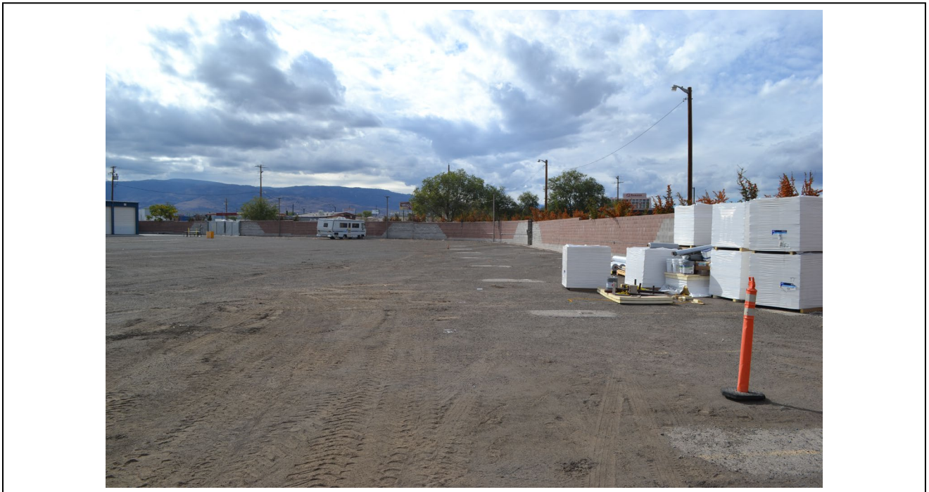
Elevation: Overview of CMU portion of Structure 2 Direction facing: 240 Photographer: S Rathbone Date: 10/25/2022
