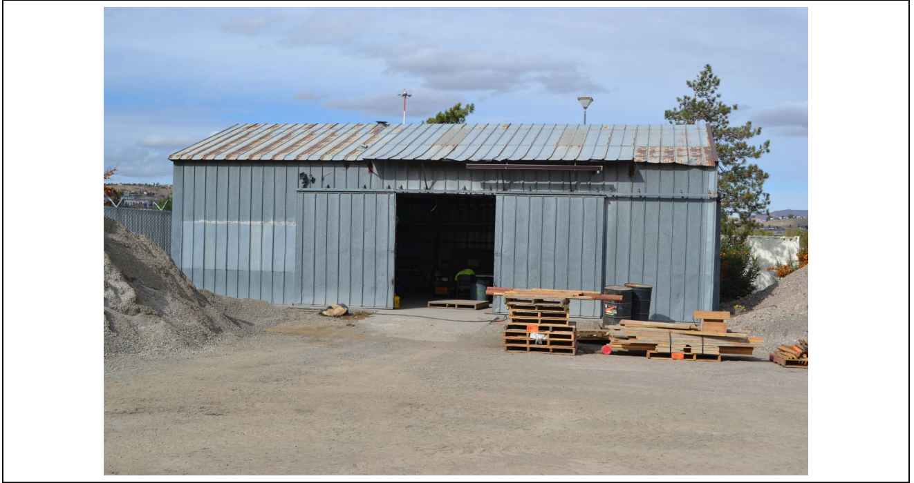
Elevation: Building 4 South elevation Date: 10/25/2022
