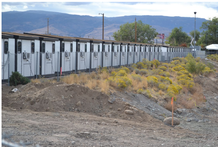
Elevation: Chain link fence on south bank of Governor's Bowl Park baseball field Direction facing: 220 Photographer: S Rathbone Date: 10/25/2022
