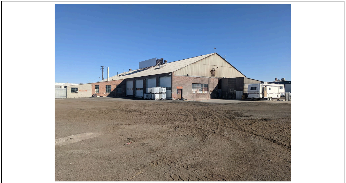
Elevation: Building 2 North west corner Date: 10/4/2022
