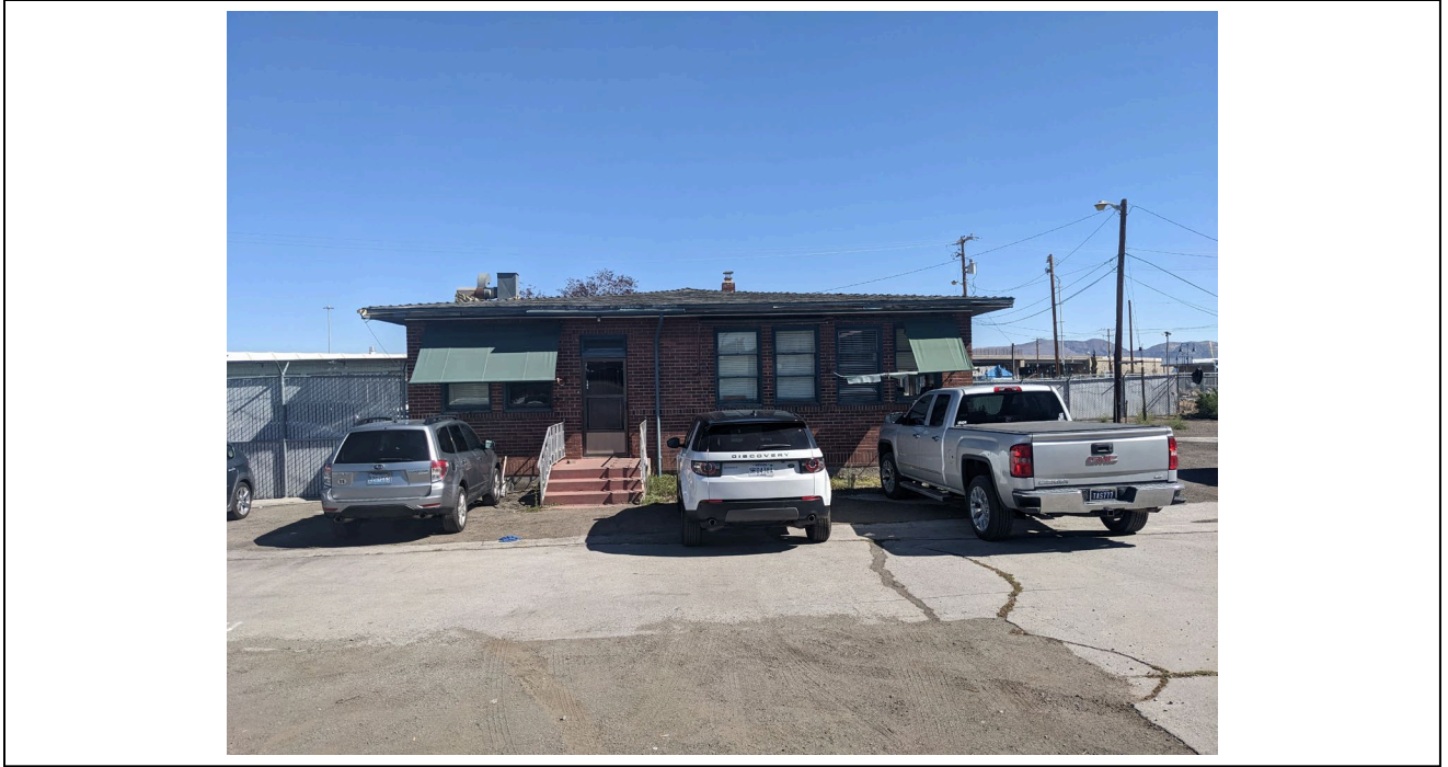
Elevation: B15585 Western elevation Direction facing: 90 Date: 10/4/2022
