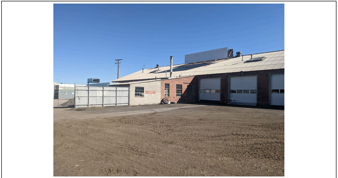
Elevation: Building 2 Boiler Room Date: 10/4/2022
