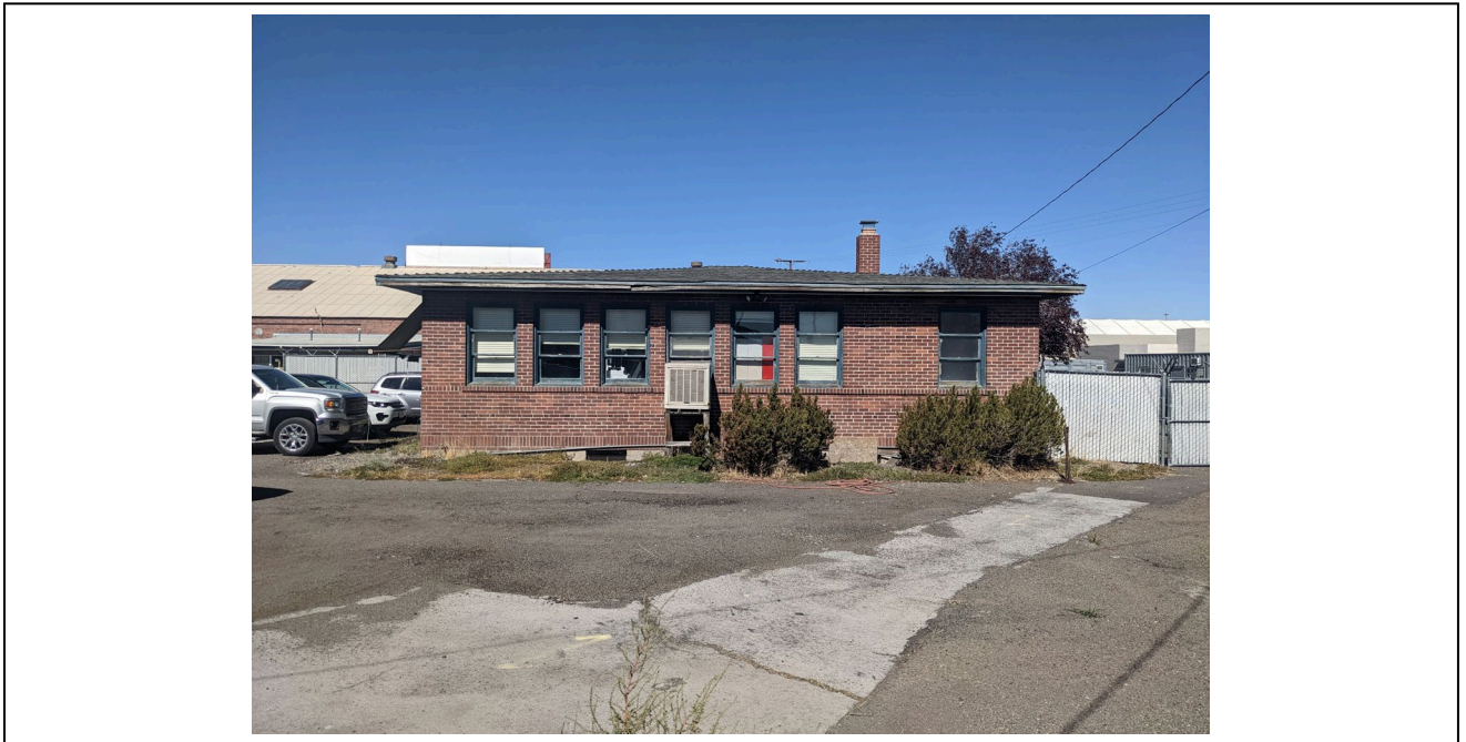
Elevation: B15585 Southern elevation Direction facing: 0 Date: 10/4/2022
