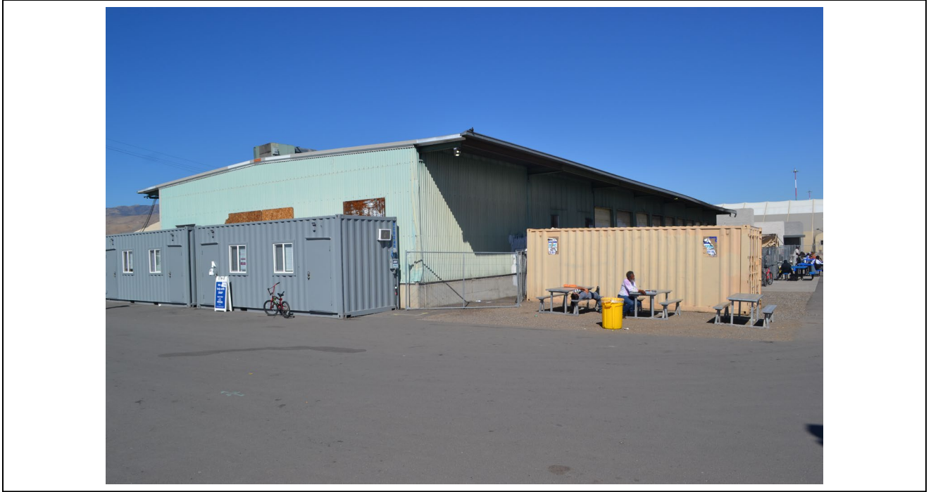
Elevation: Building 3 Southeast corner Date: 10/4/2022
