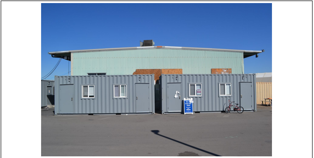
Elevation: Building 3 South elevation Date: 10/4/2022
