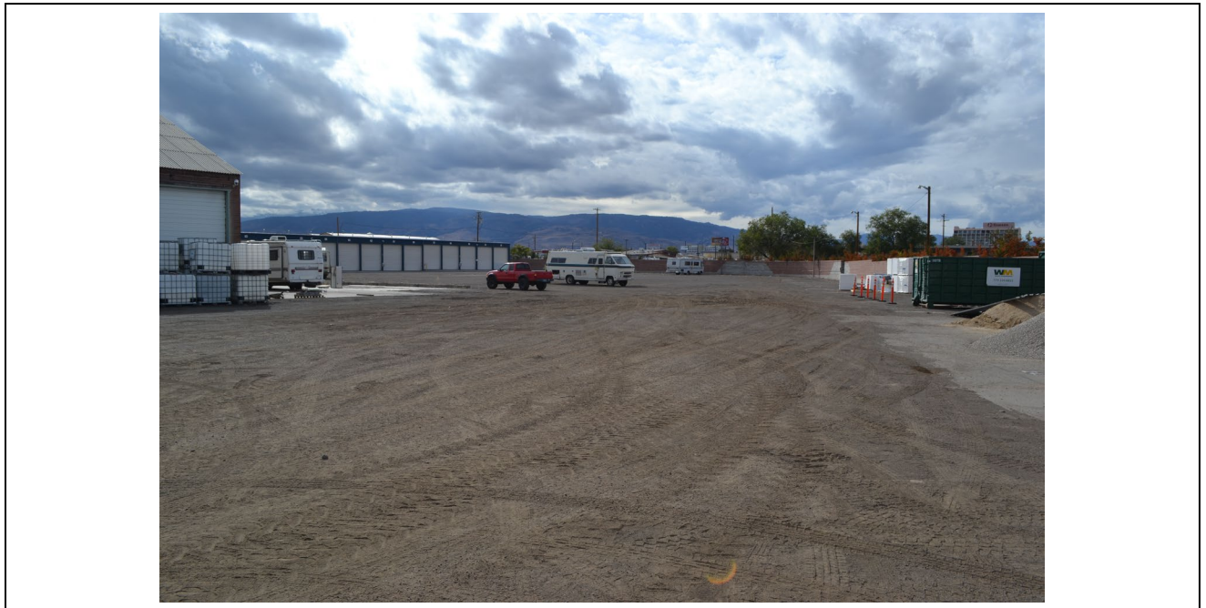
Elevation: Structure 1 Overview Date: 10/4/2022
