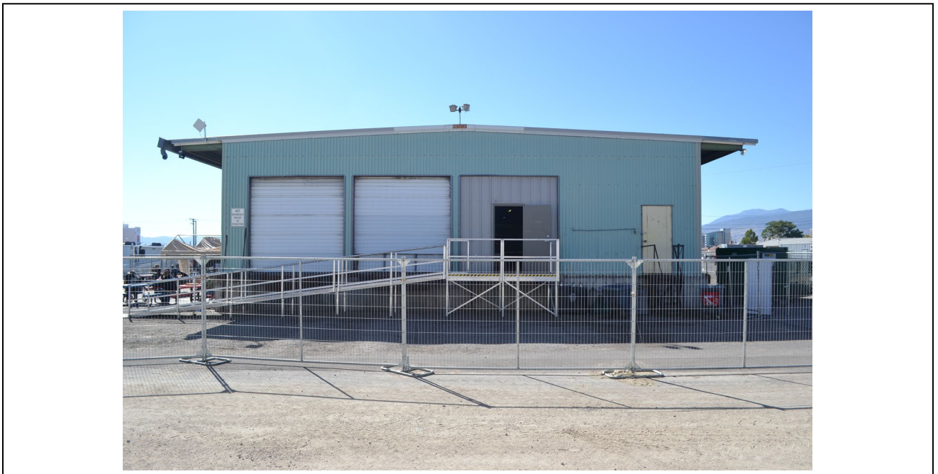
Elevation: Building 3 North elevation Direction facing: 180 Date: 10/4/2022
