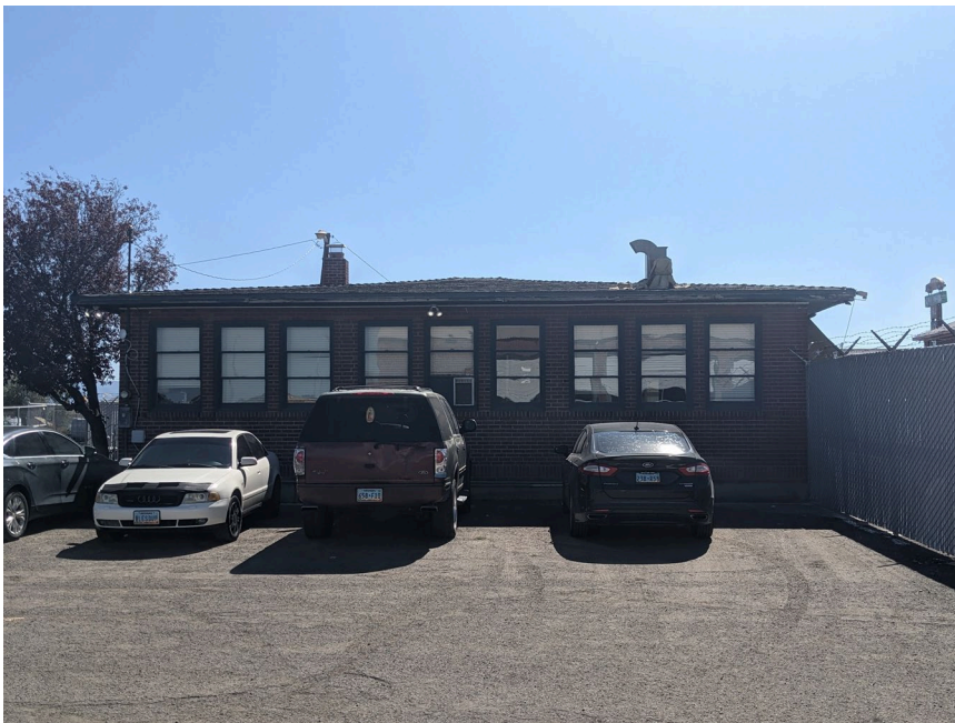
Elevation: B15585 Northern elevation Date: 10/4/2022
