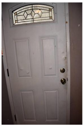
Photo: Bullet related defects to interior of front door.
