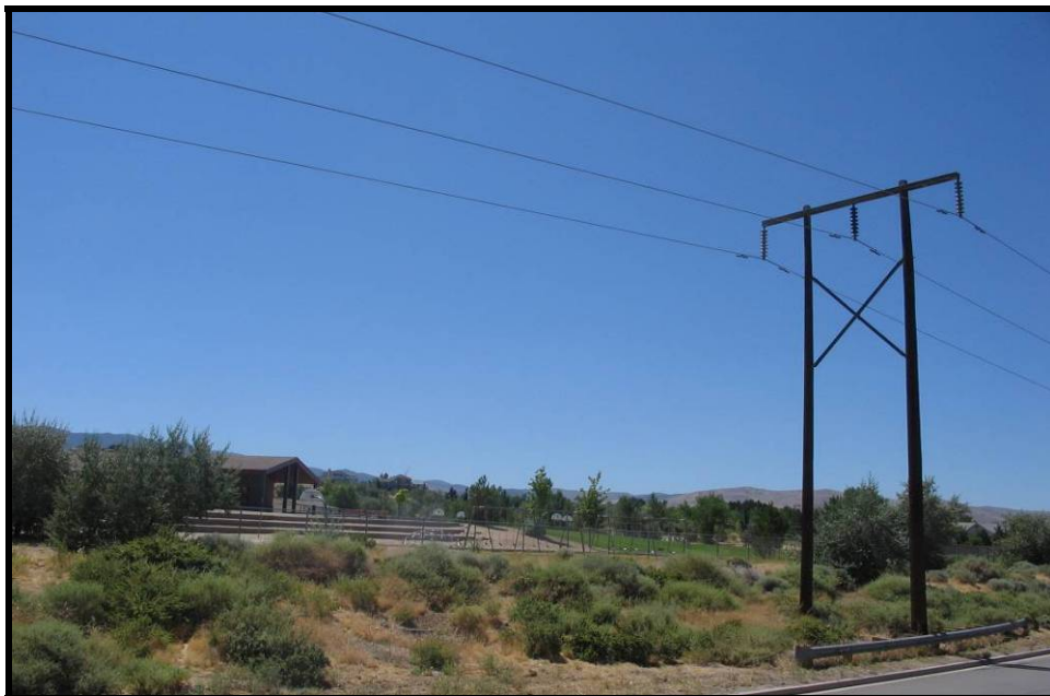
Photo 12: Transmission Line Located Adjacent to Brown Elementary School
