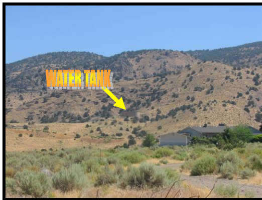
Water Tank Located at Virginia Foothills
