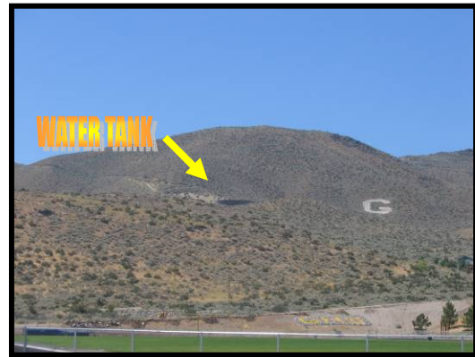
Water Tank Located in Galena
