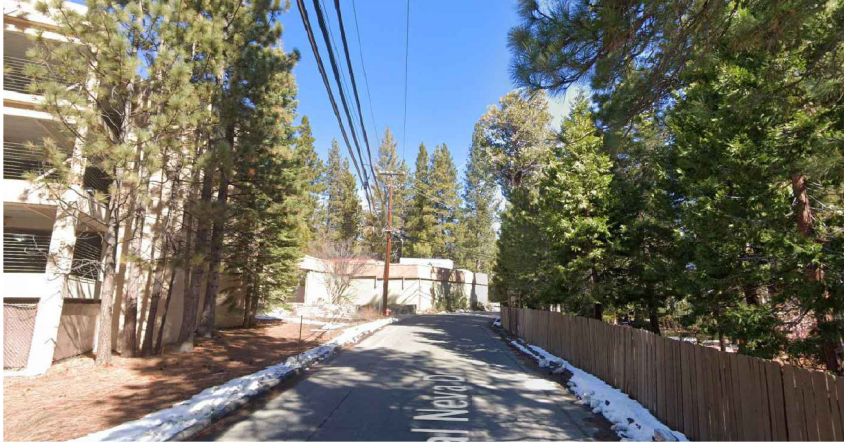
1 STREET VIEW LOOKING NORTH SHOWING TALL PARKING RAMP WALL - 3.5 STORIES TALL SOURCE: GOOGLE MAPS
