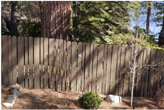
1 IMAGE OF EXISTING FENCE
