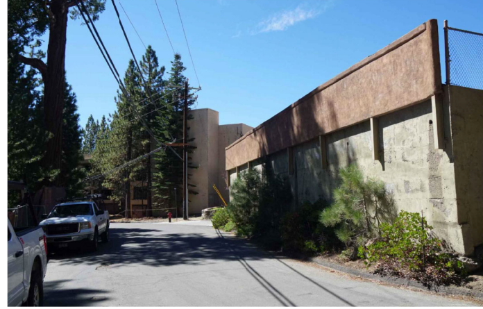
2 STREET VIEW LOOKING SOUTH SHOWING COMMERCIAL WALL & FENCE - APPX 17' TALL
