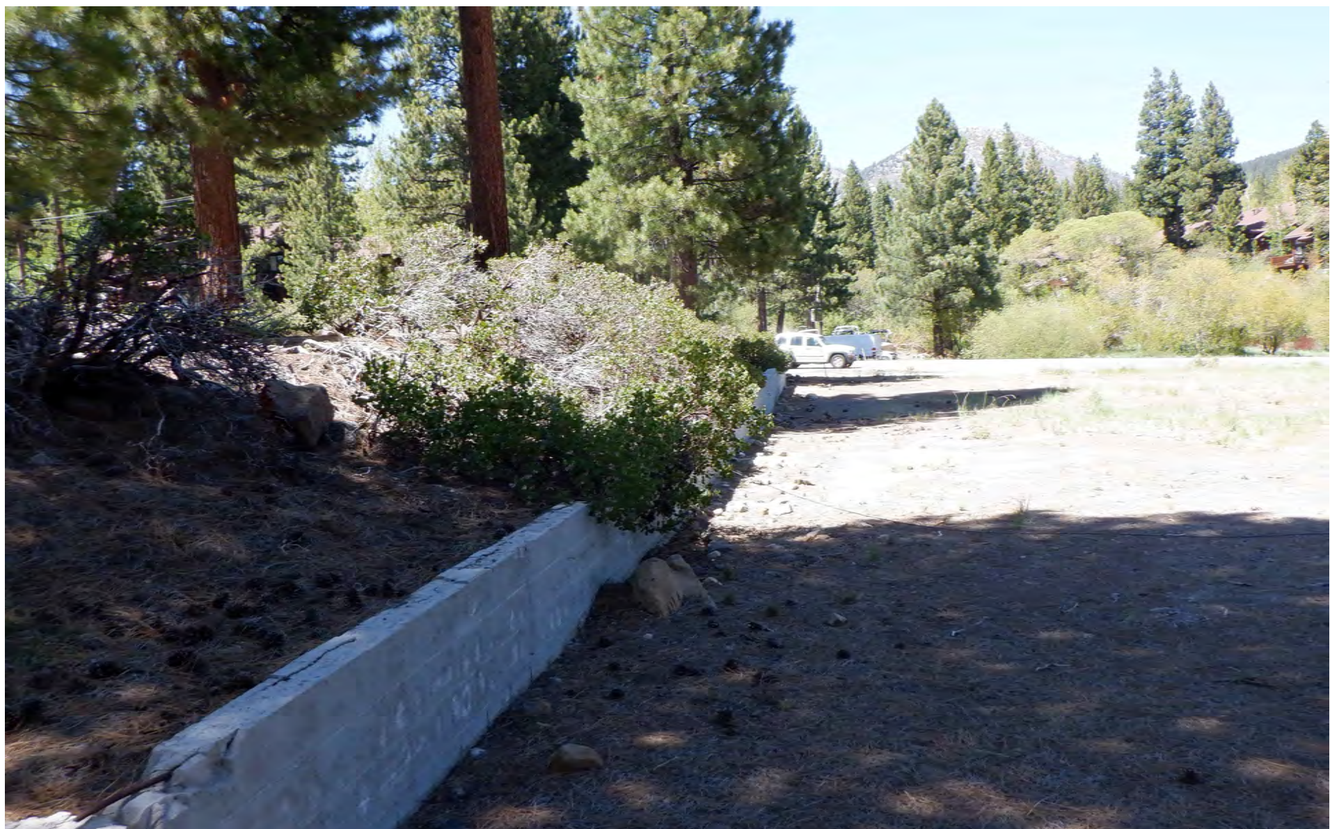
Looking North Along Retaining Wall, West Edge of Former Chevron Parcel
