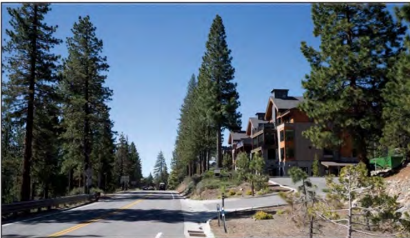
EXISTING SITE CONDITIONS
