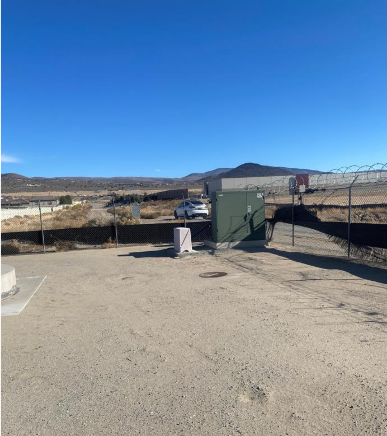
Figure 9: Example of a Similar Use Washoe County Sewer Lift Station in Spanish Springs
