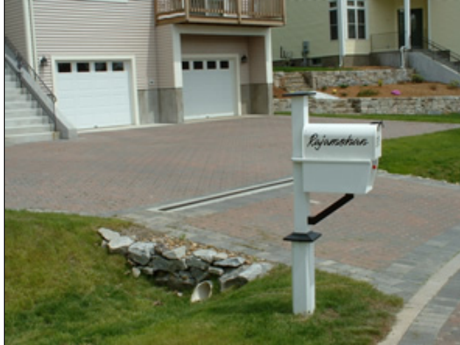
Figure 4-7. This driveway is designed with multiple LID strategies including permeable pavers and a slotted drain built in to catch sediment and runoff, which is funneled into a landscaped area. (Photo courtesy of NEMO Nevada )
