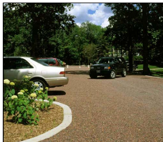
Figure 4-3. Parking grove made of a permeable paving surface. (photo from ToolBase Services )
