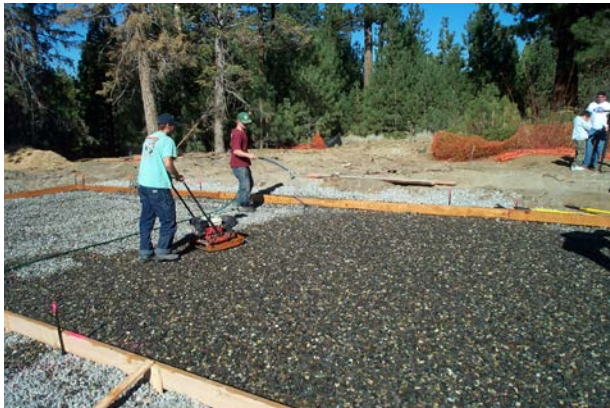
Figure 4-20. Demonstration project at Lake Tahoe. Underlying clean gravels being installed (left) and water rapidly infiltrating into porous concrete (right).
