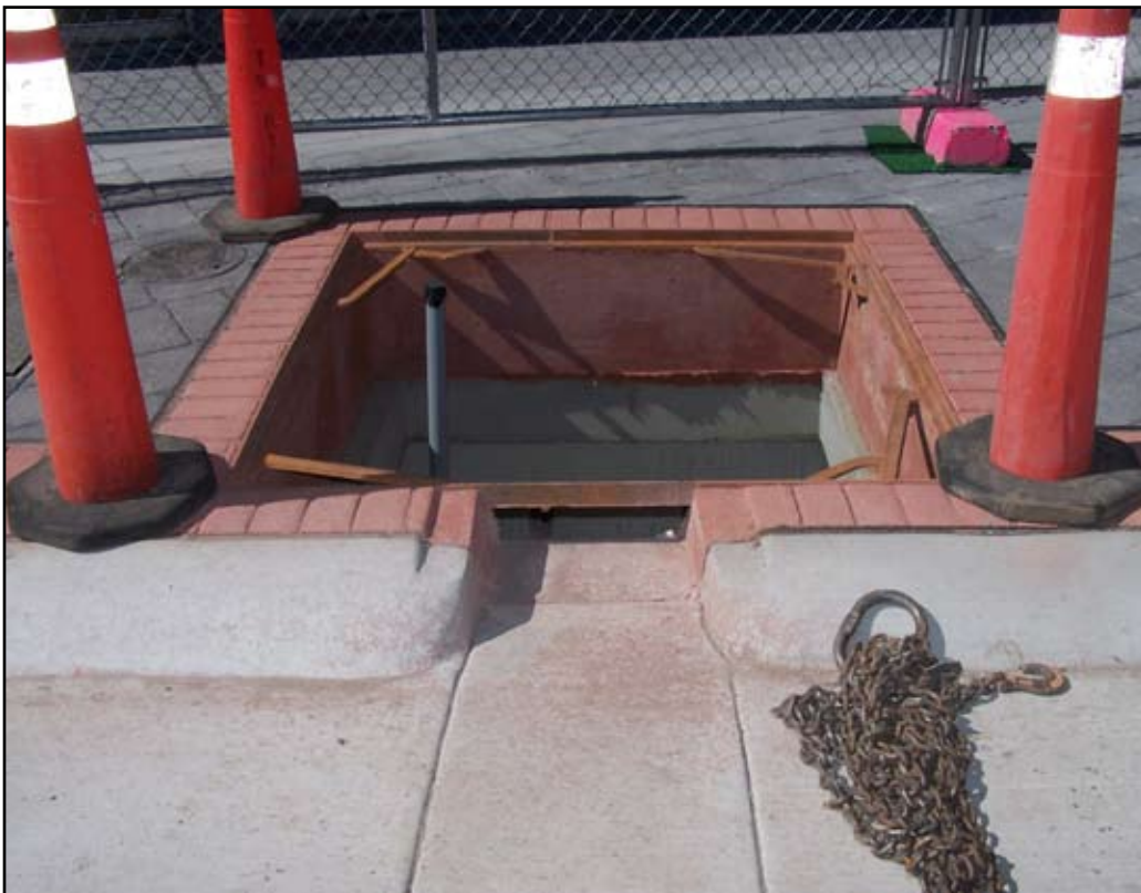
Tree filter box under construction on Virginia Street in Reno, Nevada., near the Truckee River. Runoff from the street enters the box through the curb cut.
