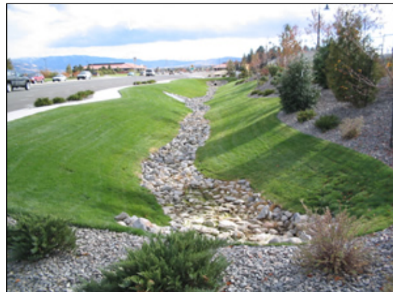
Figure 4-17. Swale with rock lined low flow channel.
