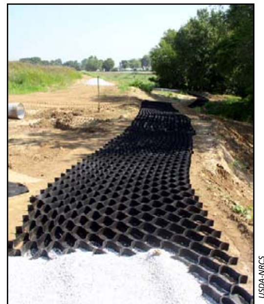
Open-celled unit pavers form the base for this graveled walking trail.
