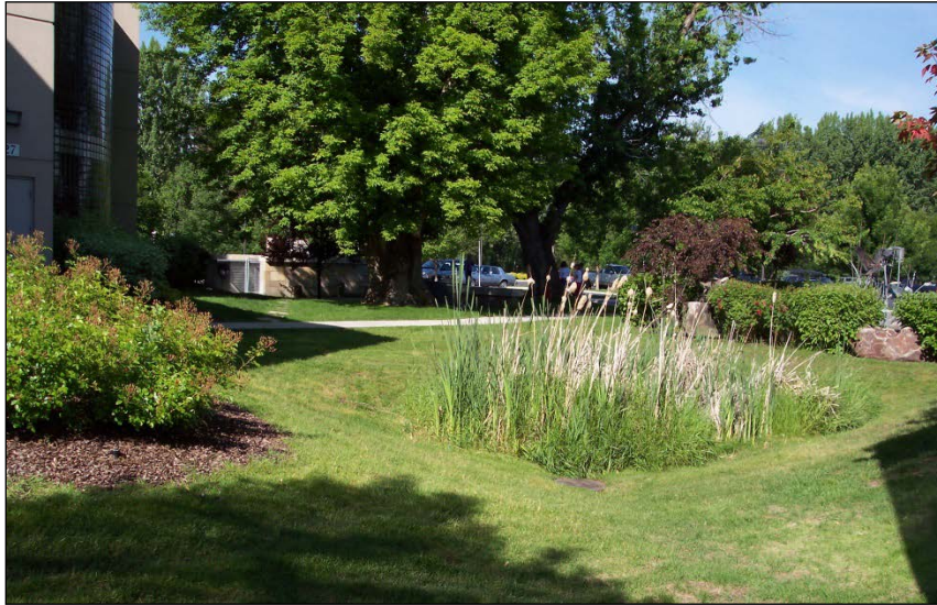
Figure 4-10. Bioretention system in a multifamily development
