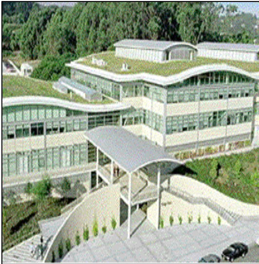
Figure 4-26. Green Roof at GAP Corporate Campus, San Bruno, CA. (Source: Rana Creek)
