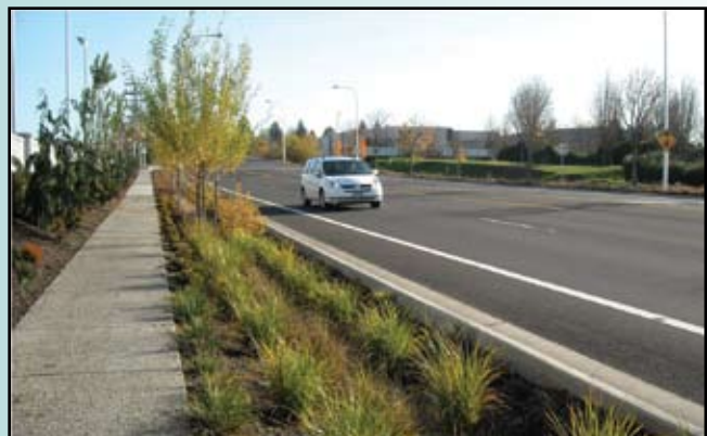
This roadside swale or bioretention basin receives and infiltrates water while providing attractive landscaping. The sidewalk made from porous concrete allows additional infiltration.
