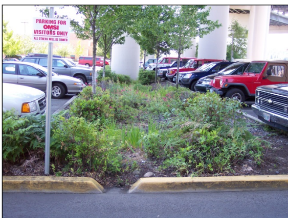
Figure 4-11. Parking lot island bioretention.
