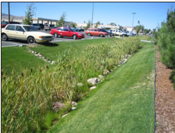
Figure 4-2. Parking lot bioretention.
