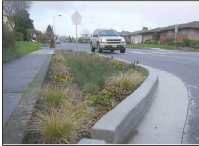
A mid-block curb extension collects stormwater runoff without requiring the removal of existing curb and gutter. Any overflow returns to the street.
