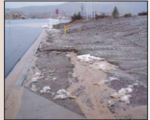
Bare slopes and impervious surfaces can result in muddy runoff that can damage rivers and streams being fed by stormwater.
