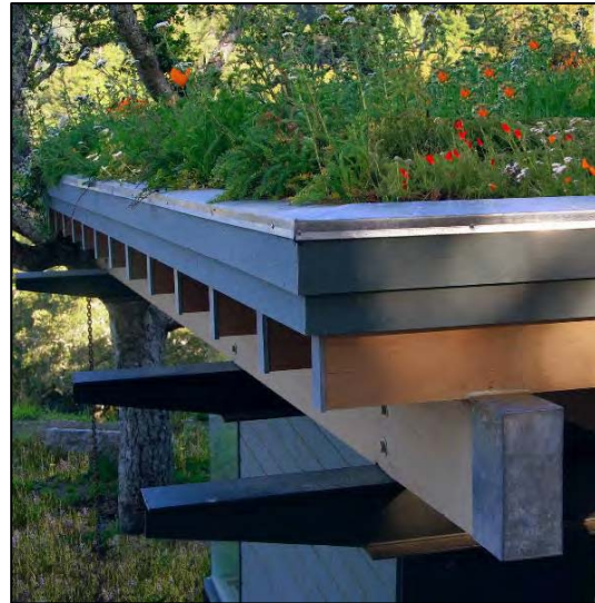
Figure 4-27. Green Roof on a commercial office building. (Source Photo: Jonathan Feldman)
