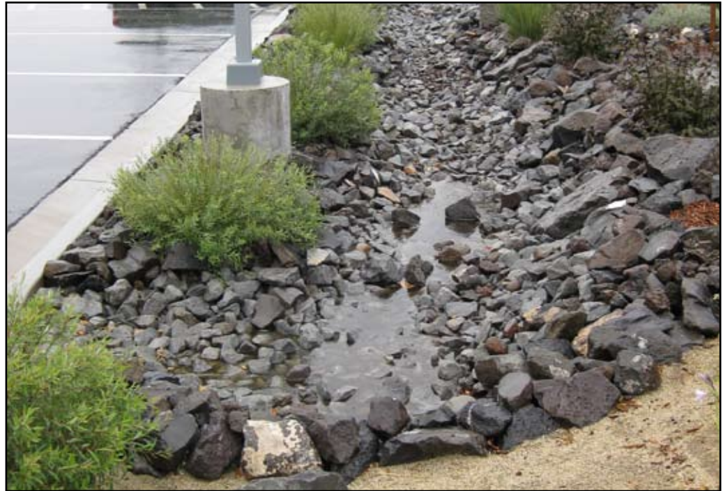
Some swales are lined with rock and have limited plant material. This makes it more difficult to remove accumulated sediment, and decreases pollutant processing by plants. Primary benefits include water retention/infiltration and sediment removal.
