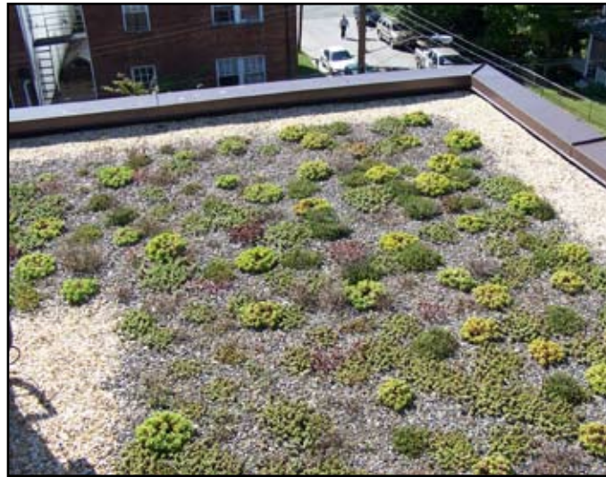
An extensive green roof planted with sedums.
