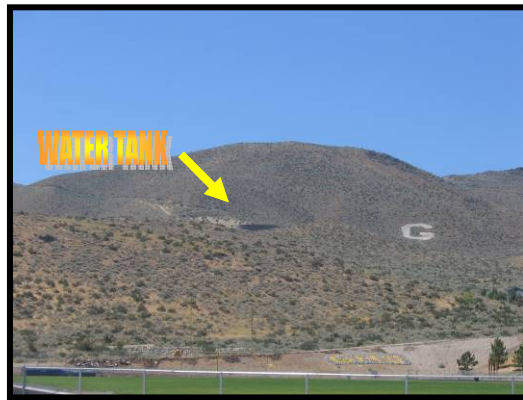
Water Tank Located in Galena
