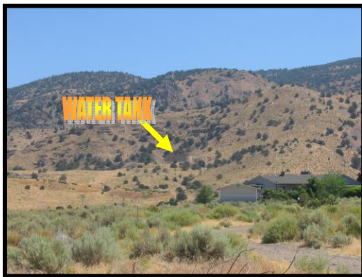
Water Tank Located at Virginia Foothills
