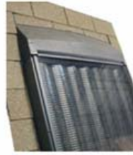
Solar Thermal Collector
