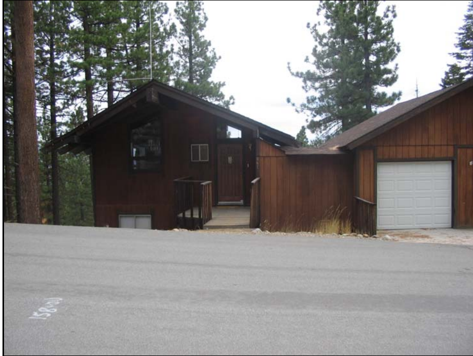
View of property looking southeast
