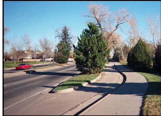
Grade separated bicycle lane, Denver, CO
