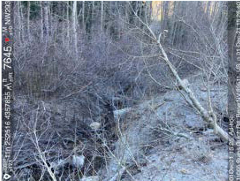
Southern edge as channel comes out of the culvert.
