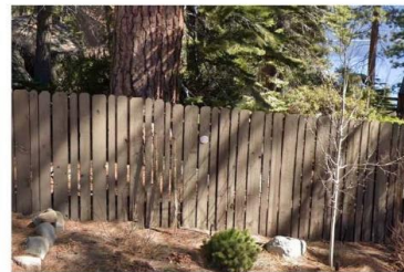
1 IMAGE OF EXISTING FENCE 1" = 1'-0" (AS SHOWN) 1/8" = 1'-0" (AS NOTED)
