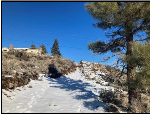
View to the north of unpermitted grading through steeper portion of site to provide safe access for percolation testing for leach field.
