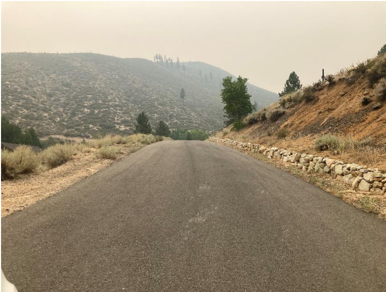
View of paved section of Bryan Canyon Road (access to the development site/pond location) – view near the northern entry to the subject parcel
