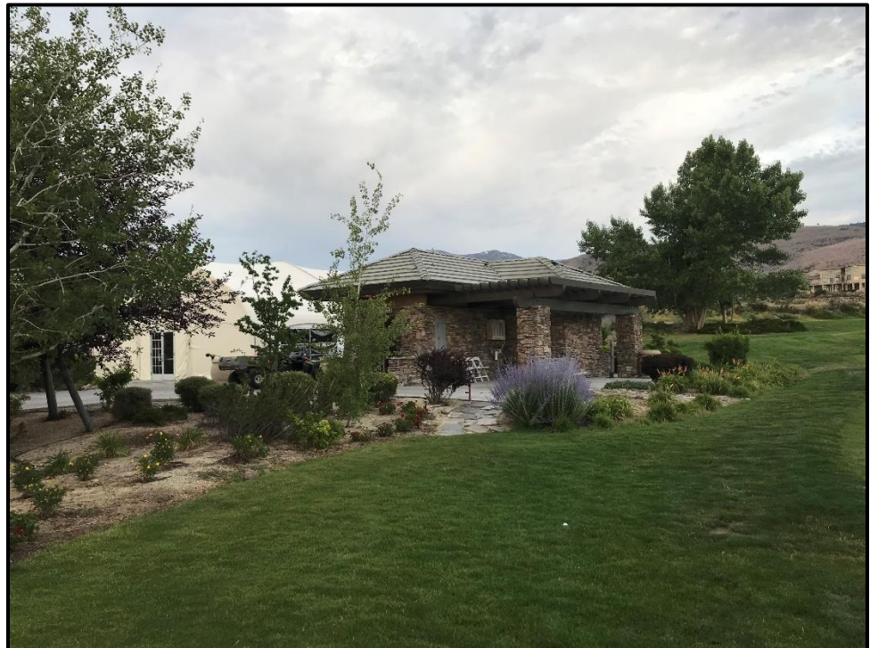
View of the existing 9- Iron concession building (to remain after new construction)
