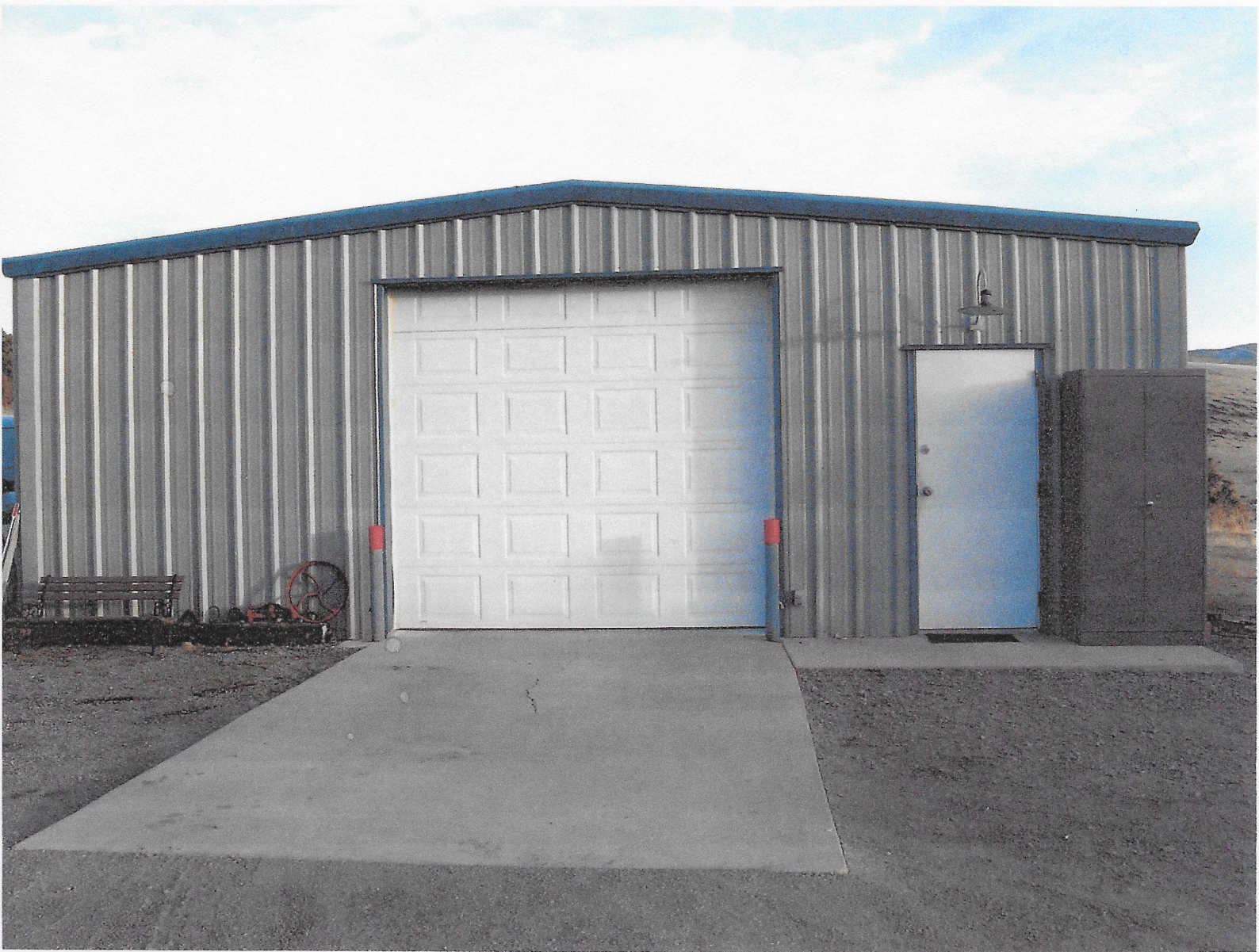
ATTACHMENT #3. Looking east at the west end of the existing metal building
