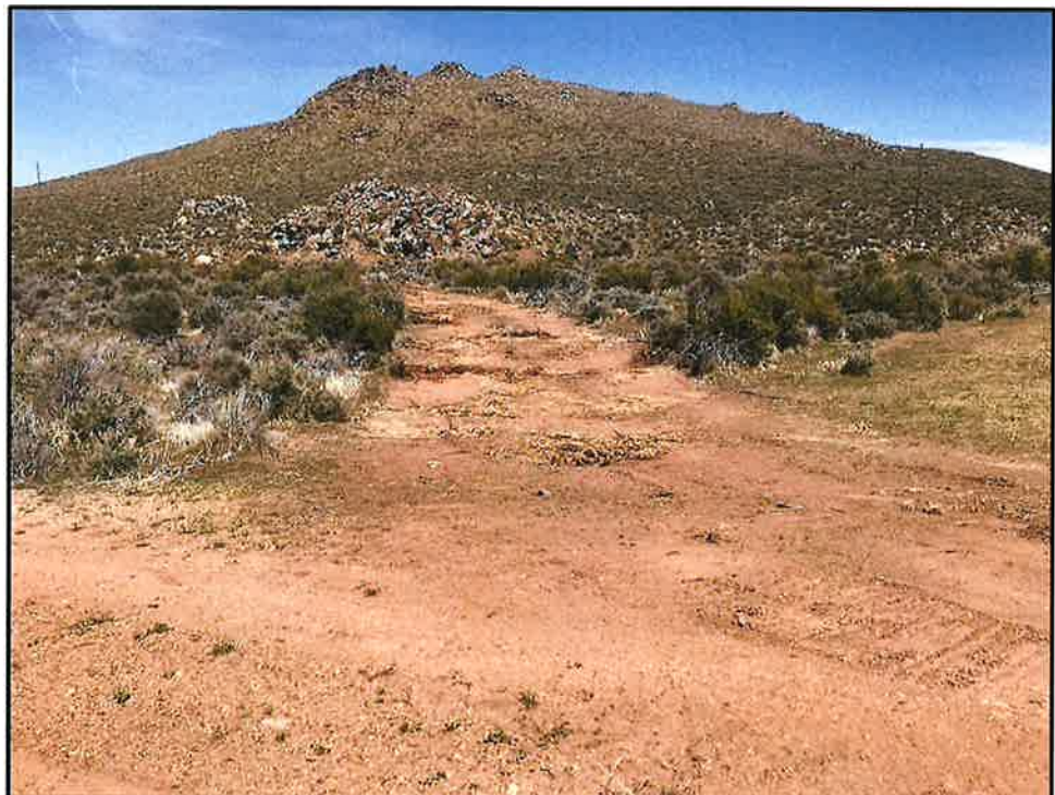
Portion of new access that branches off of existing sewer line road where vegetation was crushed, but earth was not "regraded."
