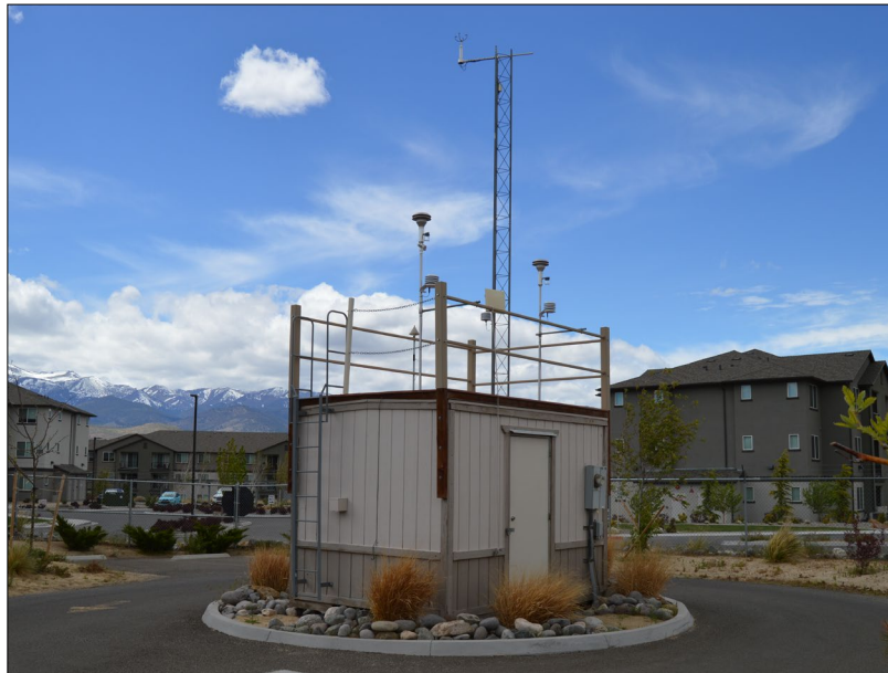
Figure 16 Toll Monitoring Station
