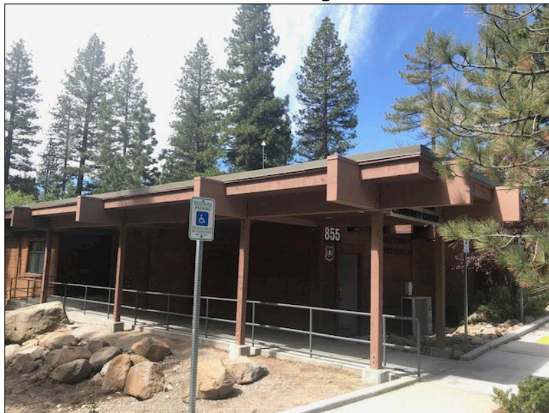
Figure 4 Incline Monitoring Station
