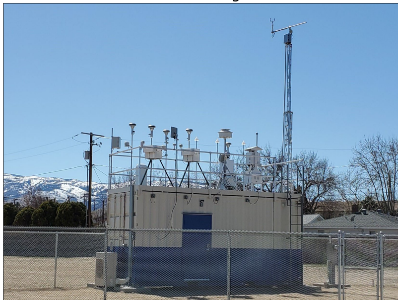
Figure 8 Reno4 Monitoring Station
