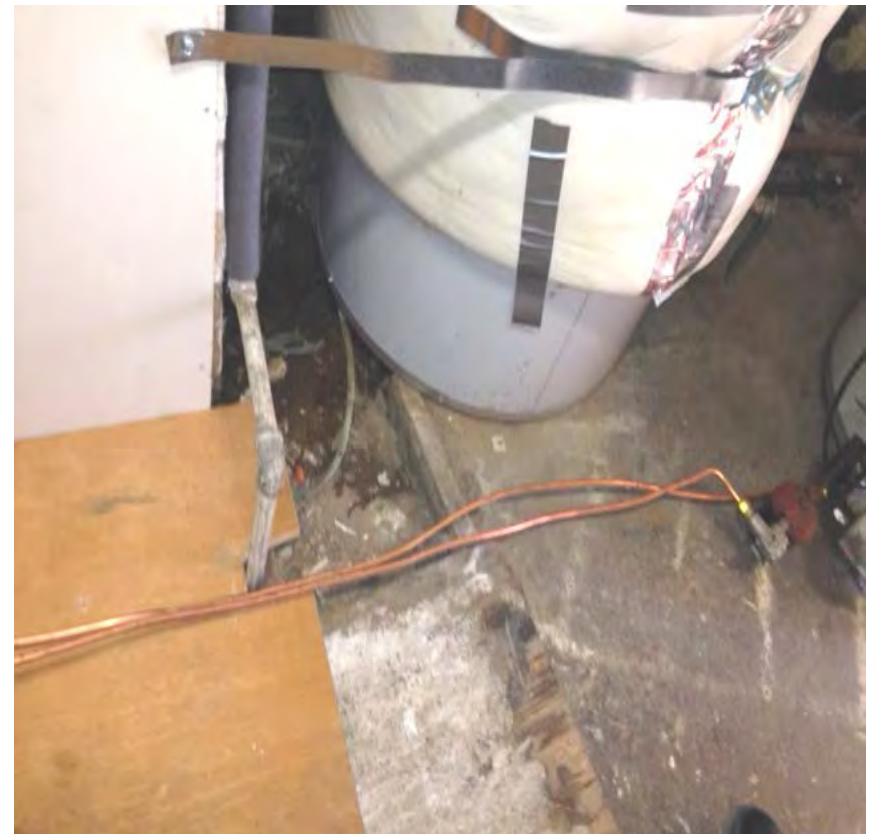
Kerosene fed into furnace 15' away
