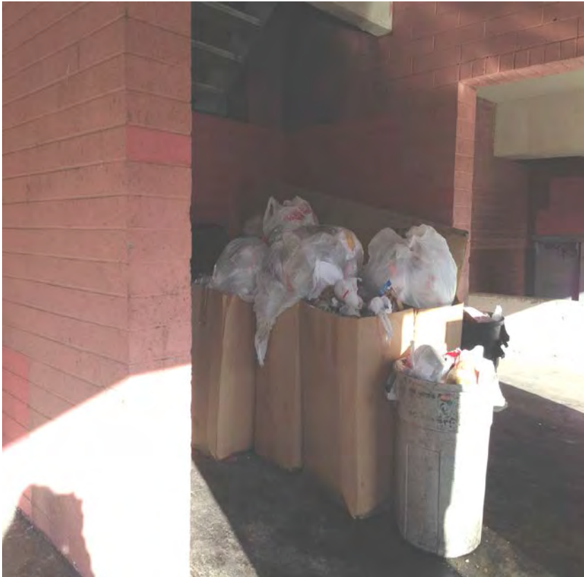
Improper Waste Storage
