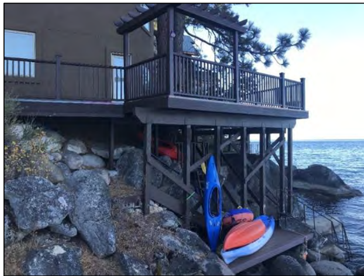
Applicant's Stairs and Deck Built in the ROW
