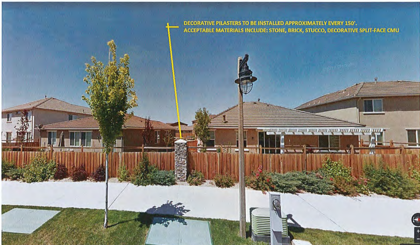
Figure 15 – Typical Silver Hills Parkway Fencing
