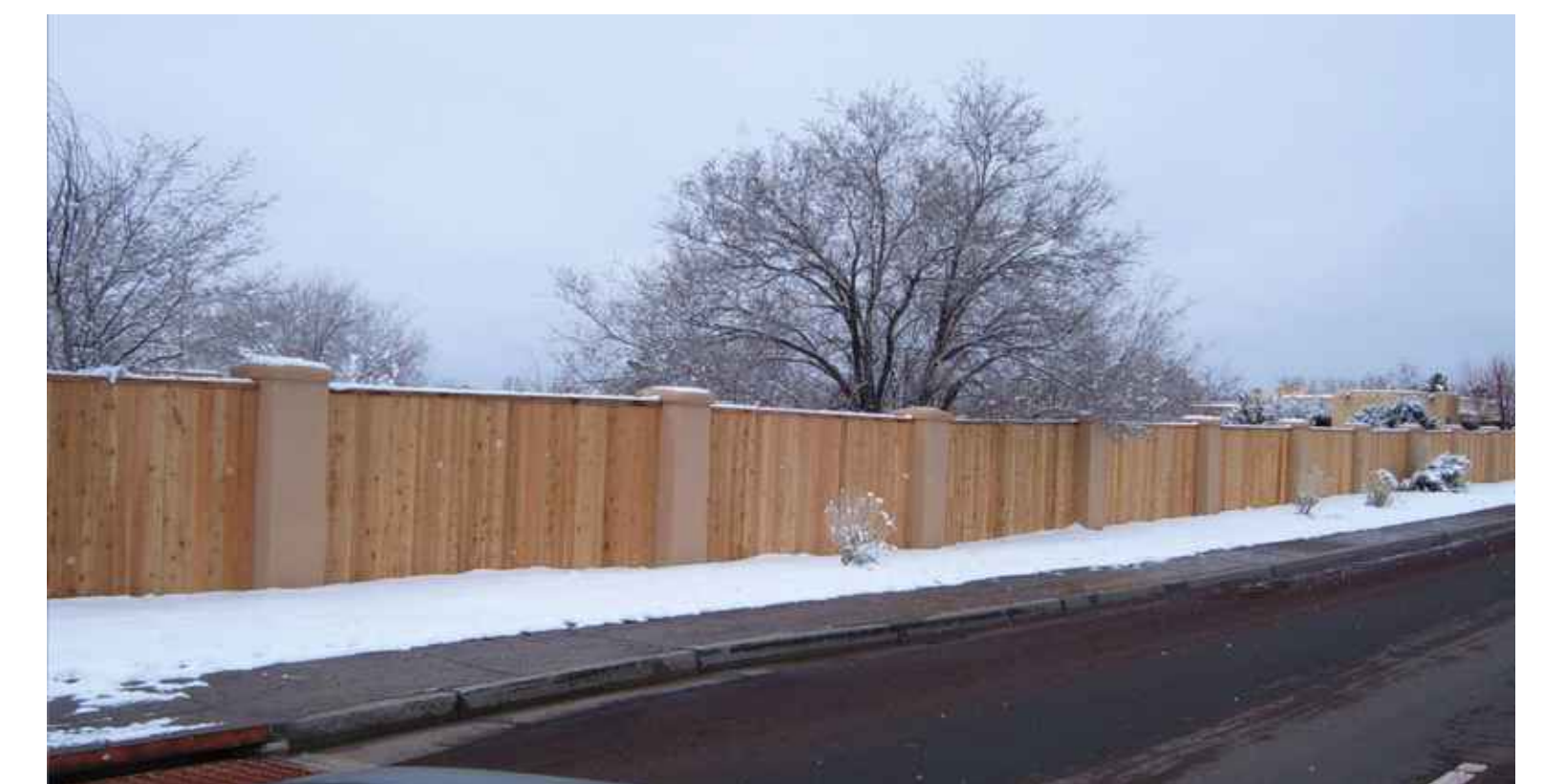
FENCING WITH PILASTERS ALONG MT. ROSE HWY
