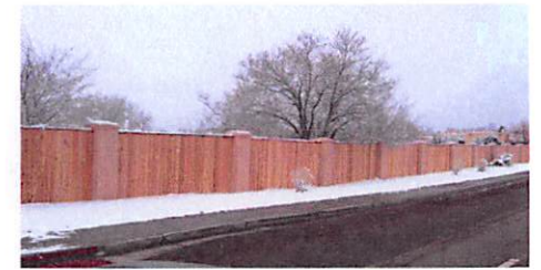
FENCING WITH PILASTERS ALONG MT. ROSE HWY
