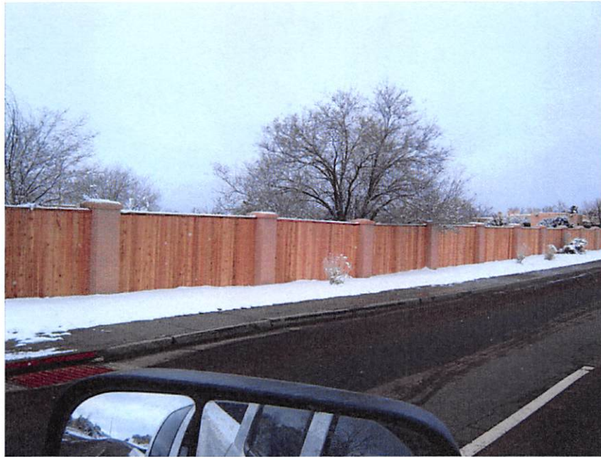
Fencing along Mt Rose Highway
