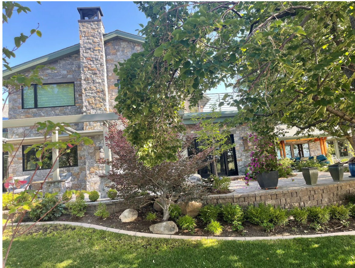
SOUTH VIEW LIVING AREA AND UPPER FLOOR
