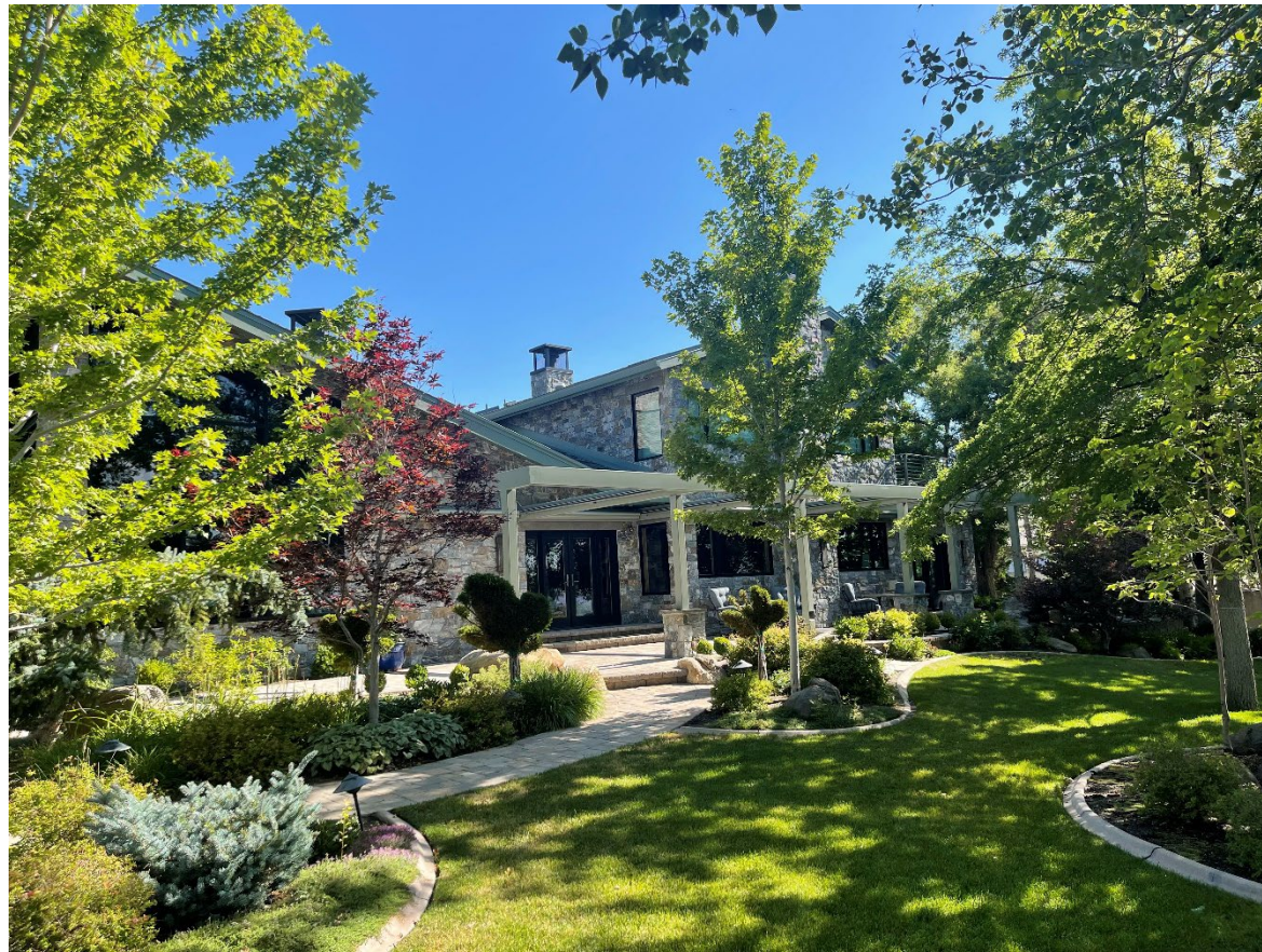
SOUTH VIEW EXTERIOR PATIO STRUCTURE
