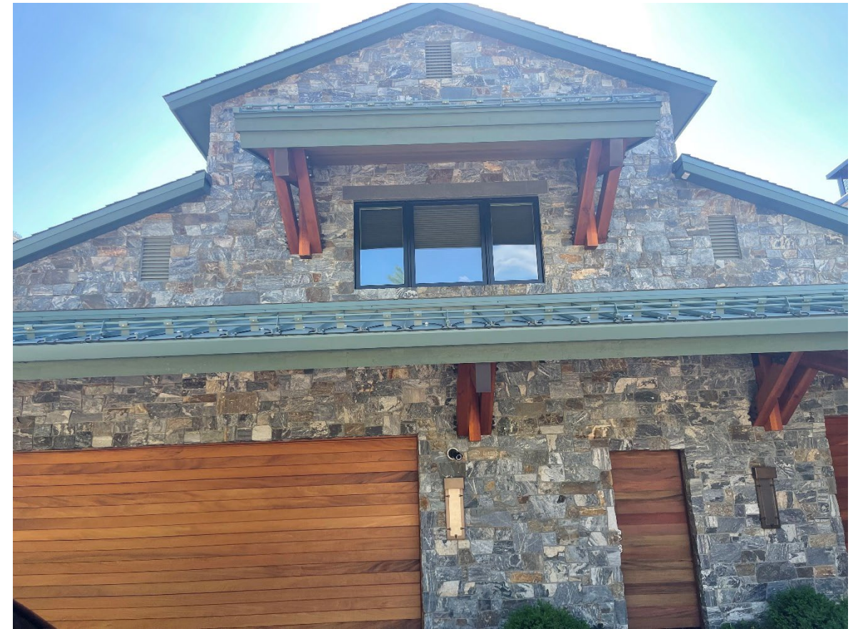
WEST VIEW AT GARAGE LOWER ROOF TRANSITION TO BREEZEWAY / ROOF CANOPY
