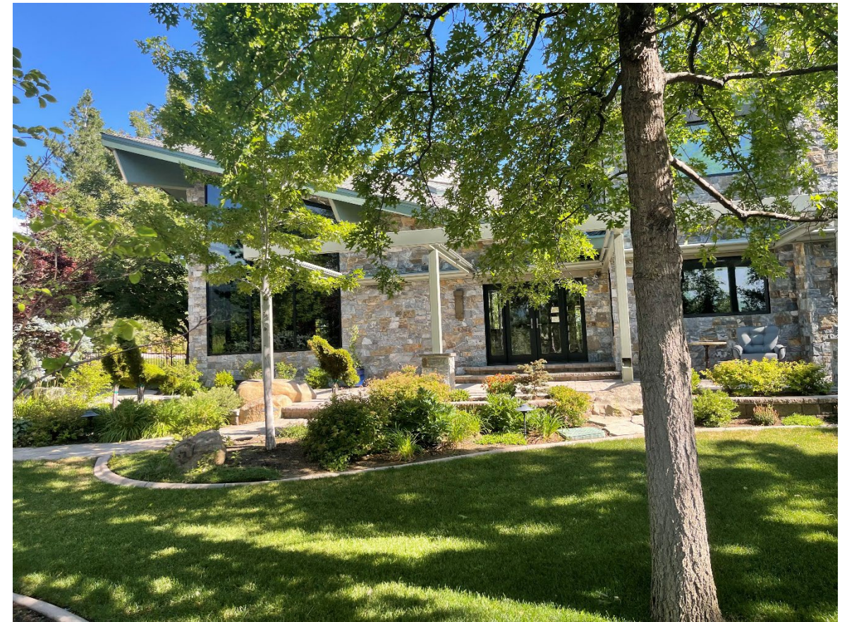
SOUTH VIEW GREATROOM & EXTERIOR PATIO STRUCTURE TRANSITION
