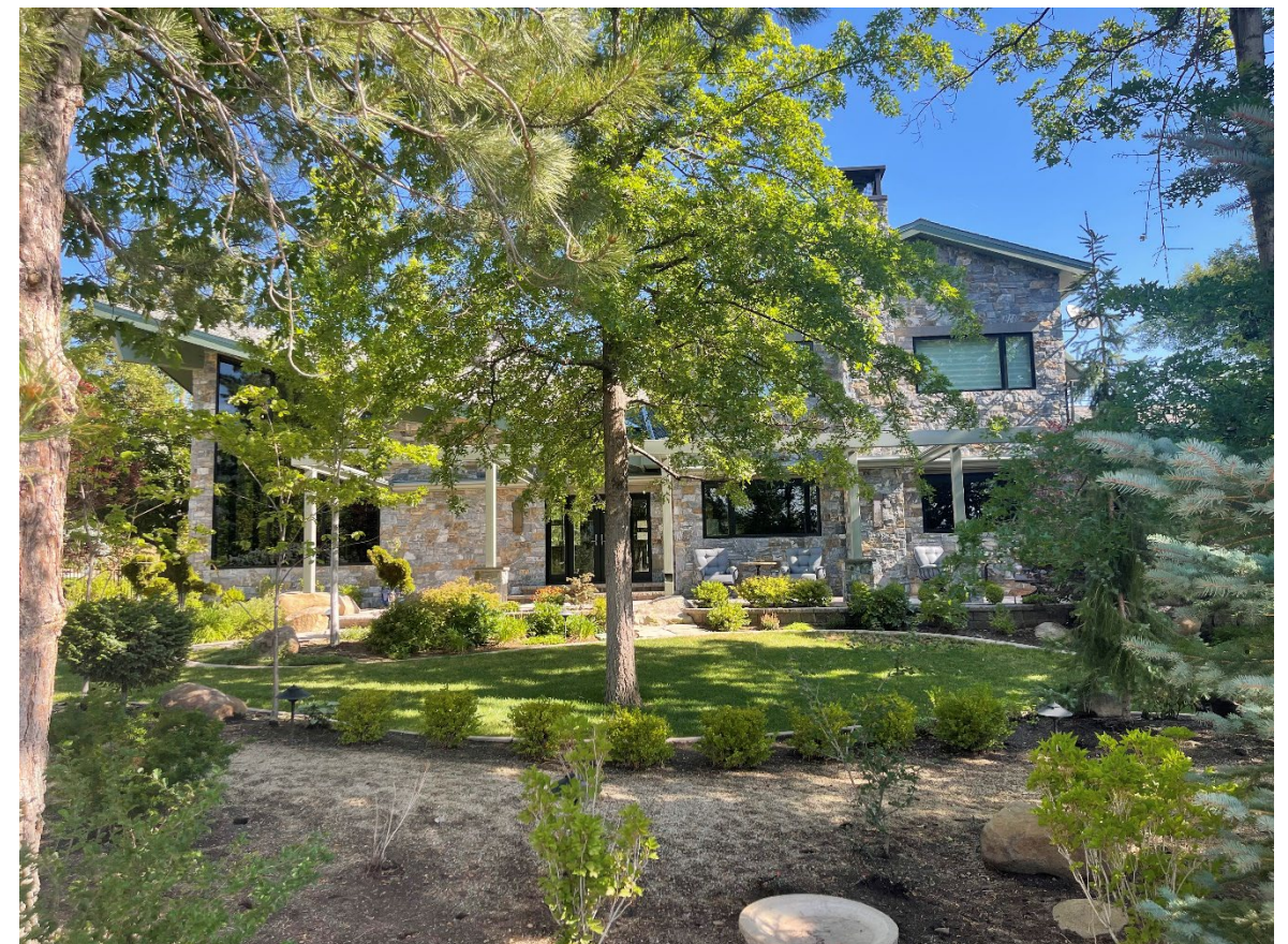
SOUTH VIEW GREATROOM TO PATIO STRUCTURE TRANSITION AND UPPER FLOOR
