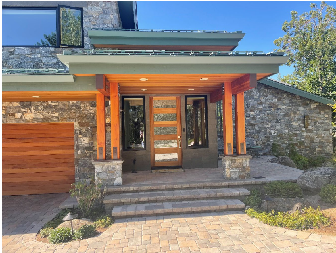
NORTH VIEW PRIMARY RESIDENCE ENTRY
