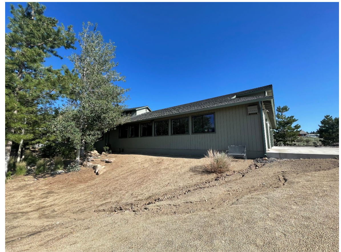
SOUTH VIEW AT GARAGE
