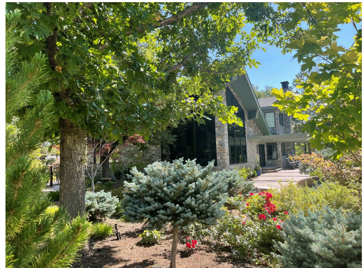
SOUTHWEST VIEW AT GREATROOM AND EXTERIOR PATIO STRUCTURE
