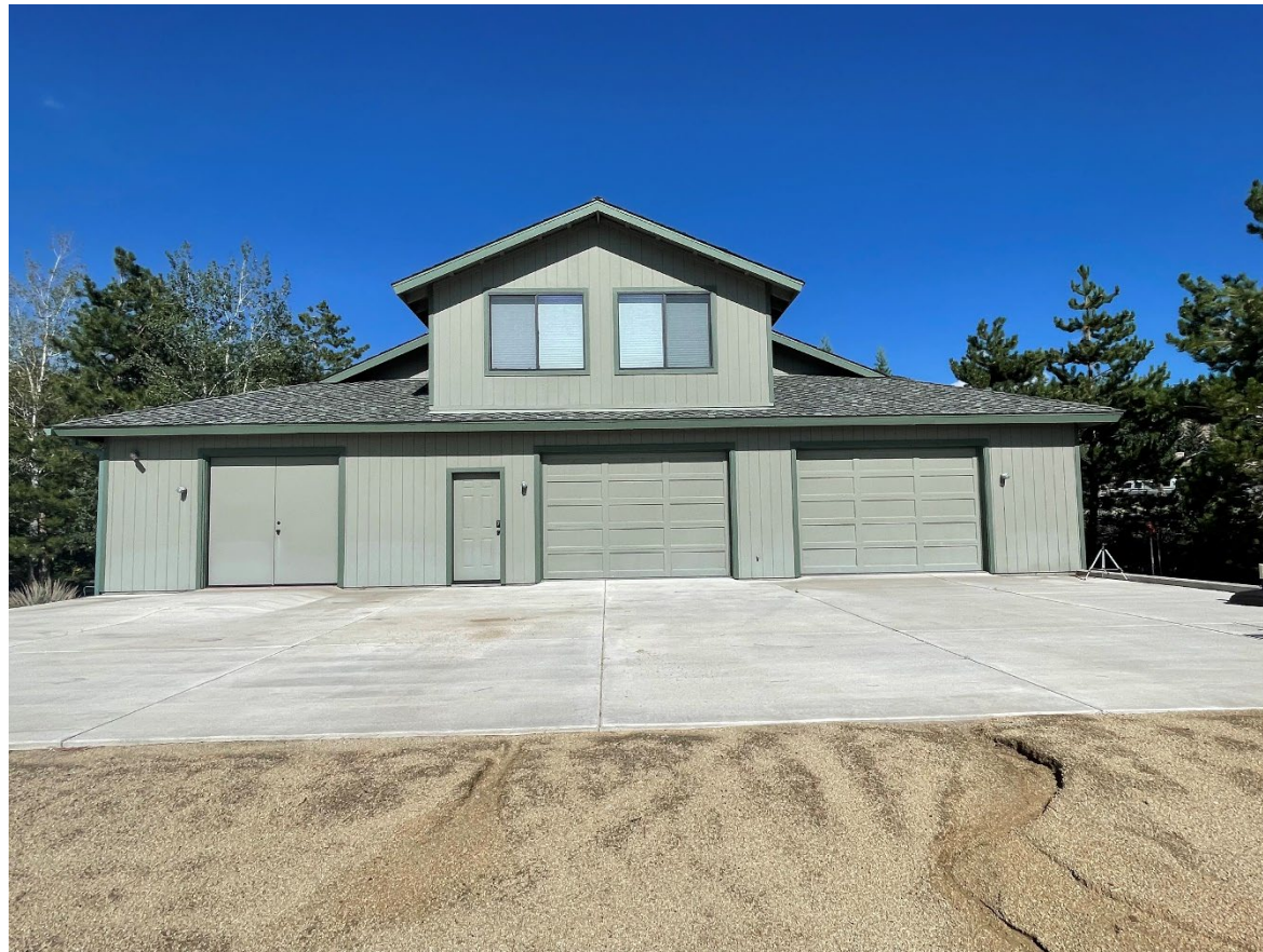
EAST VIEW GARAGE - NORTH VIEW INACCESSIBLE TO PHOTOGRAPH DUE TO ADJOINING PROPERTY PROXIMITY. NORTH VIEW AT GARAGE SIMILAR TO SOUTH VIEW
