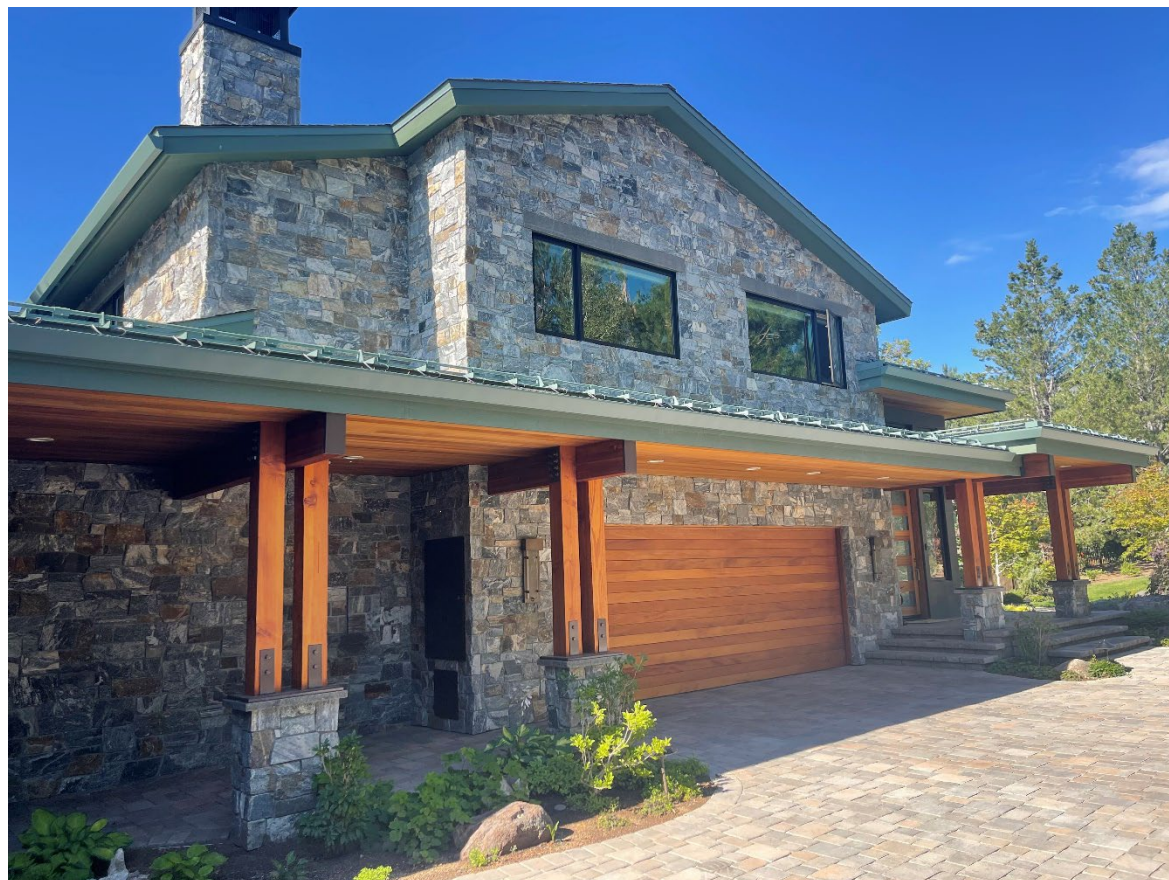
NORTH VIEW PRIMARY RESIDENCE & BREEZEWAY / ROOF CANOPY TOWARDS ENTRY
