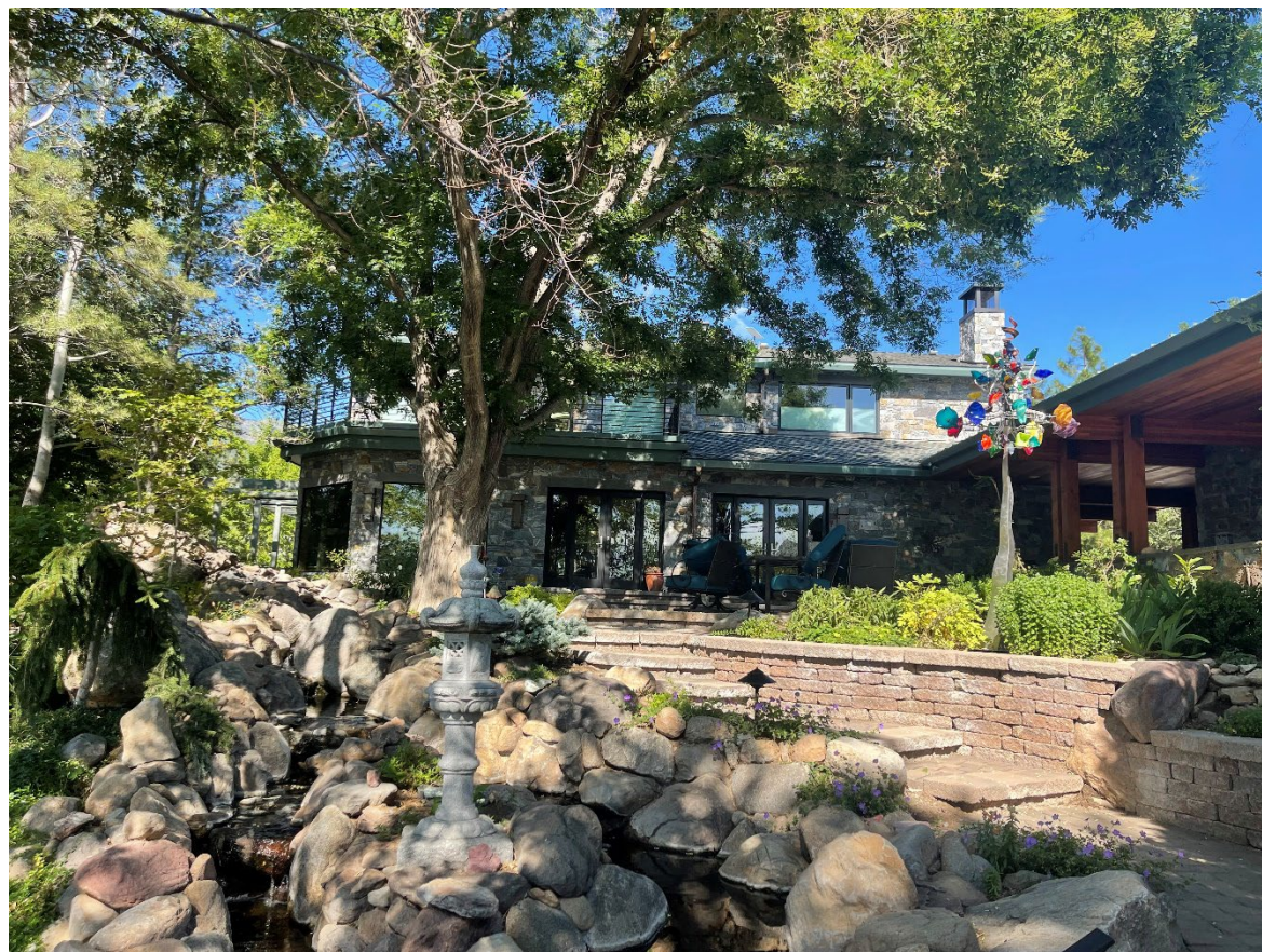
EAST VIEW LIVING AREA AND UPPER FLOOR BALCONY TRANSITION
