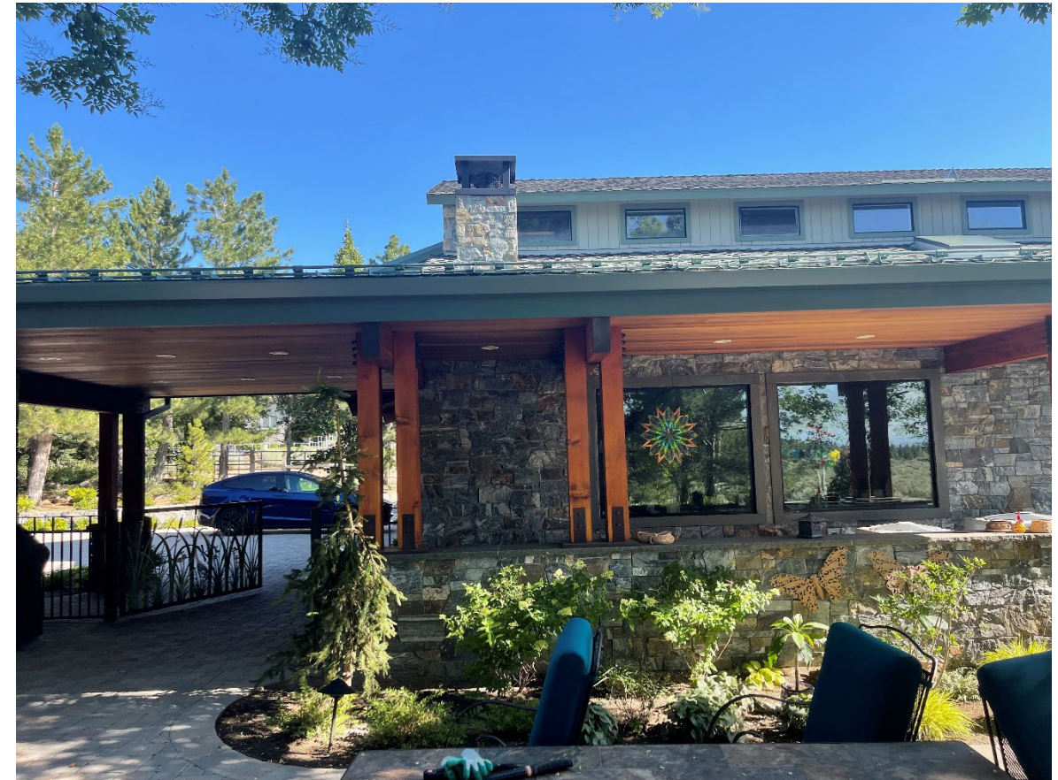
SOUTH VIEW GARAGE TO BREEZEWAY / ROOF CANOPY TRANSITION
