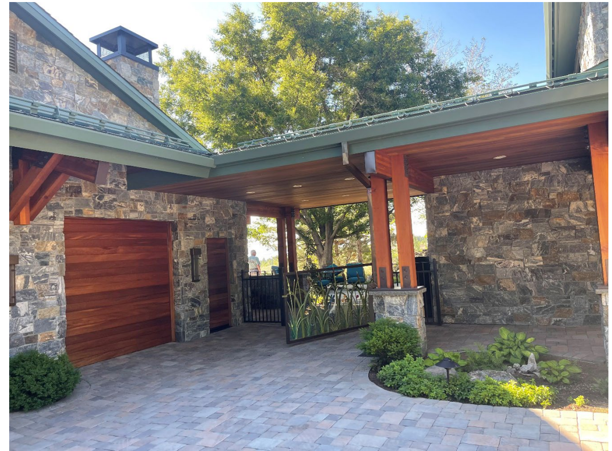
NORTHEAST GARAGE & PRIMARY RESIDENCE OPEN BREEZEWAY / ROOF CANOPY
