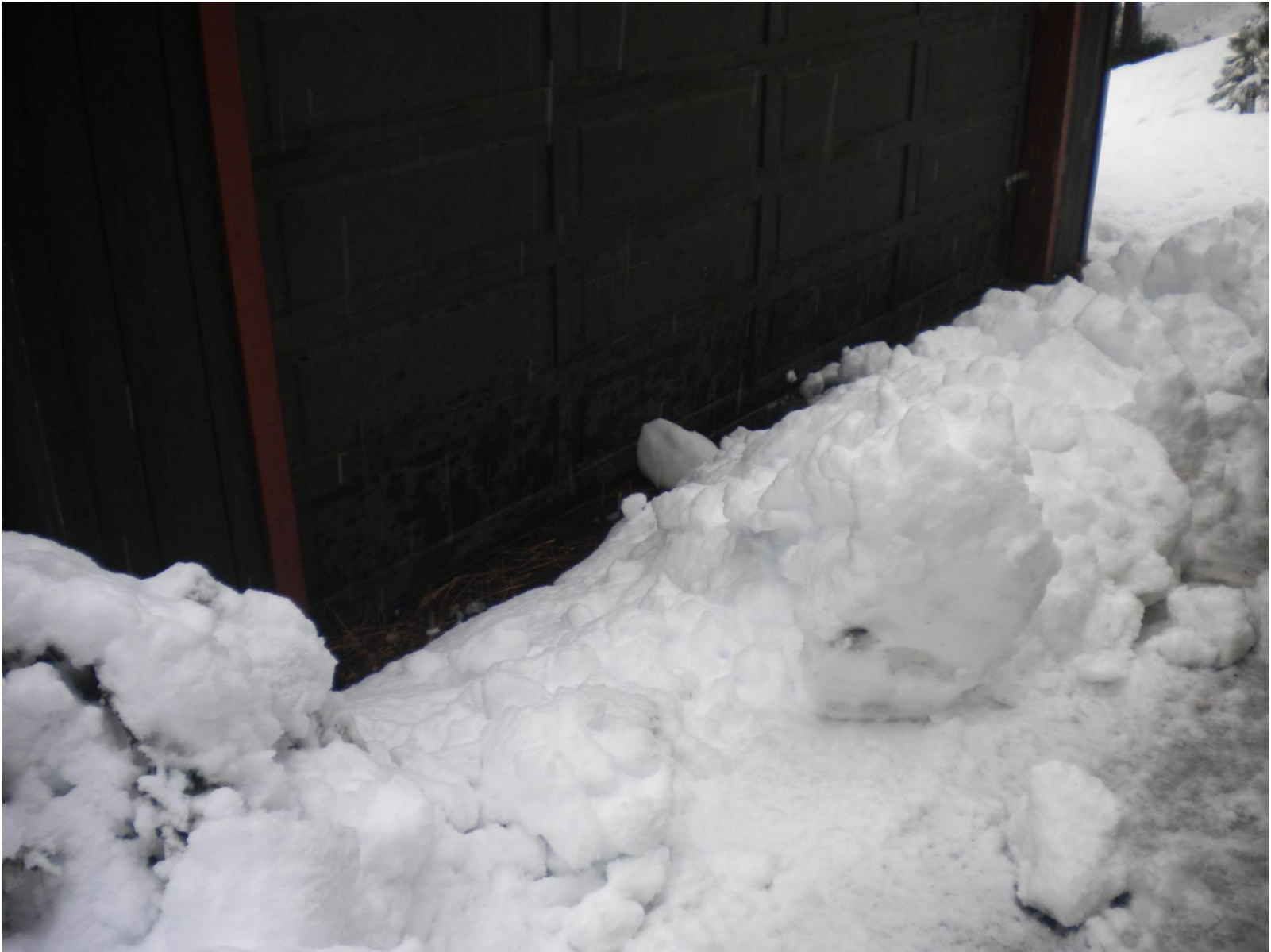
Picture #6 – Standing on the edge of the Tuscarora rd. looking at steep entrance to garage with snow conditions.
