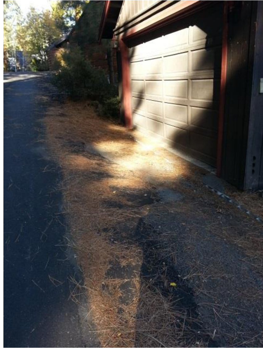
Picture #2 – Grade break at garage looking north on Tuscarora rd.
