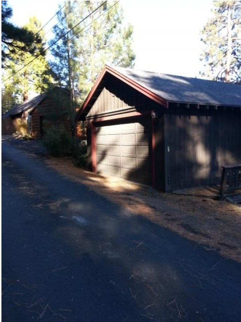
Picture #1 – Garage looking north on Tuscarora rd.
