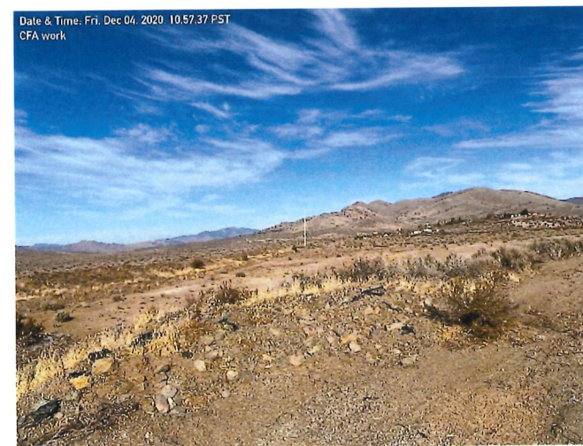
Photo from the southwest corner of the site, along Reno Park Boulevard toward the north. Existing drop-off from Reno Park Boulevard to the primary portion of the site can be seen in the foreground.
