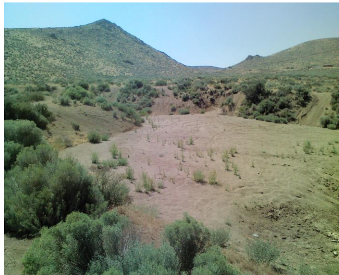
Large Excavation in the South Parcel
